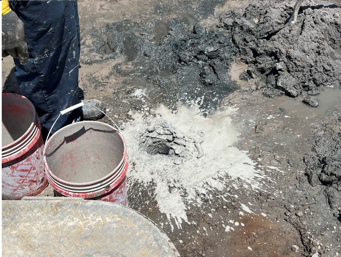
Photo 2- Representative photo of GES grouting a coring location.
