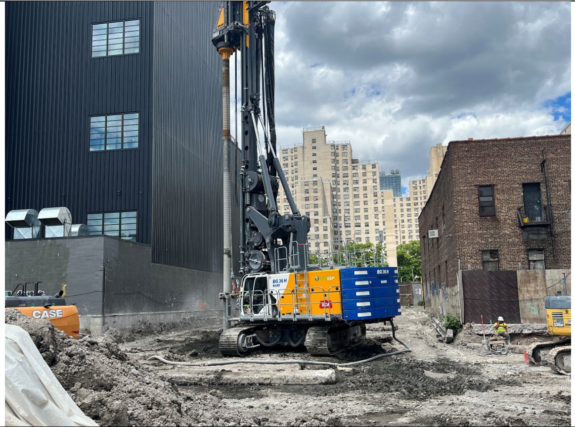
Photo 3- Representative photo of ISS column installation.
