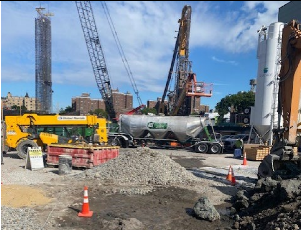
Photo 1- Representative photo of a delivery of slag.
