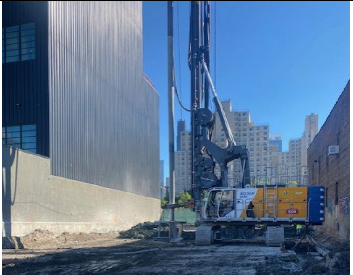
Photo 3- Representative photo of ISS column installation.
