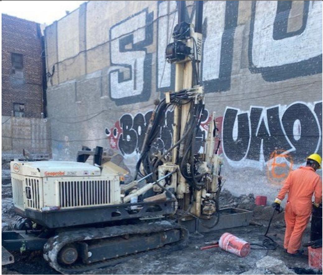
Photo 2- Representative photo of GES and MTL conducting geo-technical drilling.
