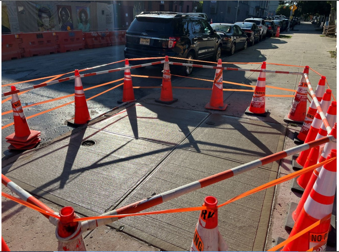
Photo 1- Representative photo of completed national grid work.
