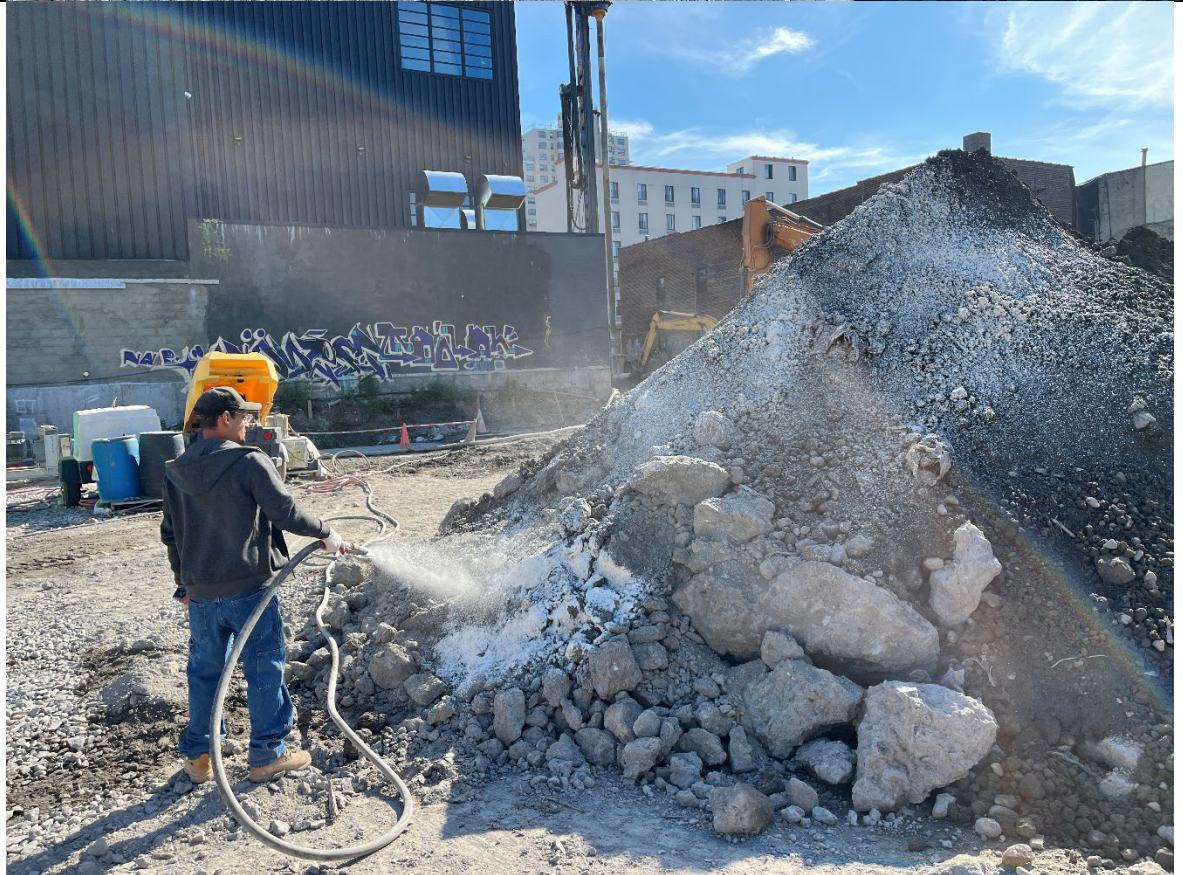
Photo 2- Representative photo of ATMOS foam sprayed over swell stockpile.
