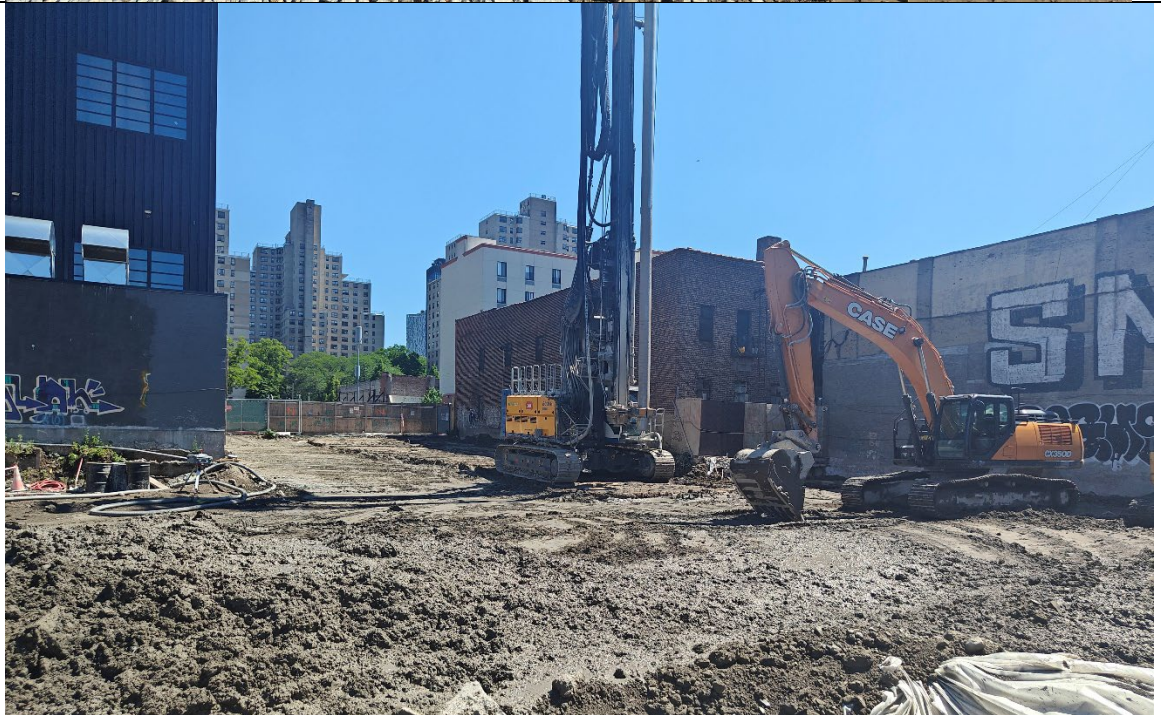
Photo 2- Representative photo of site at the end of the days activities.
