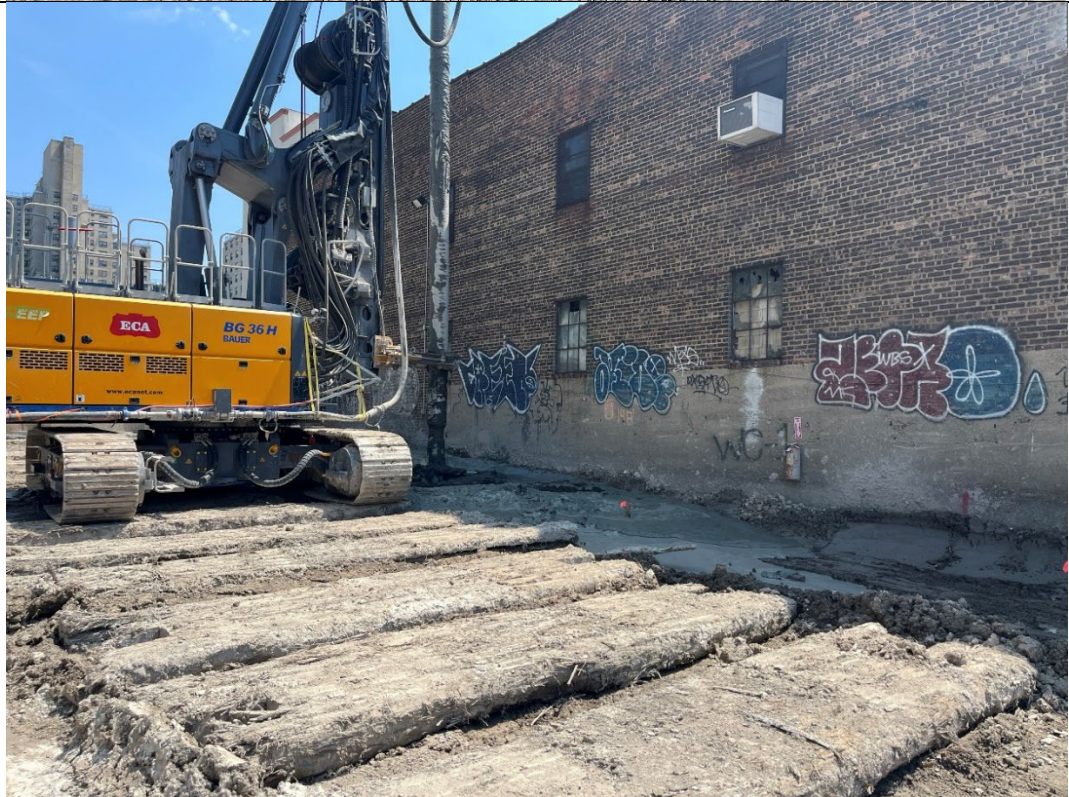
Photo 2- Representative photo of ISS Column installation.
