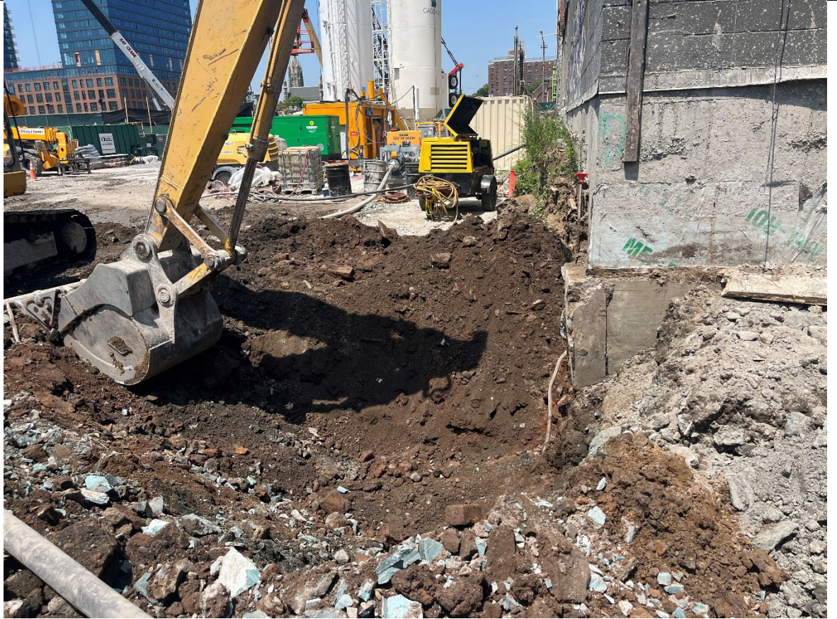
Photo 4- Representative photo of obstruction removal in southwestern portion of the alley.
