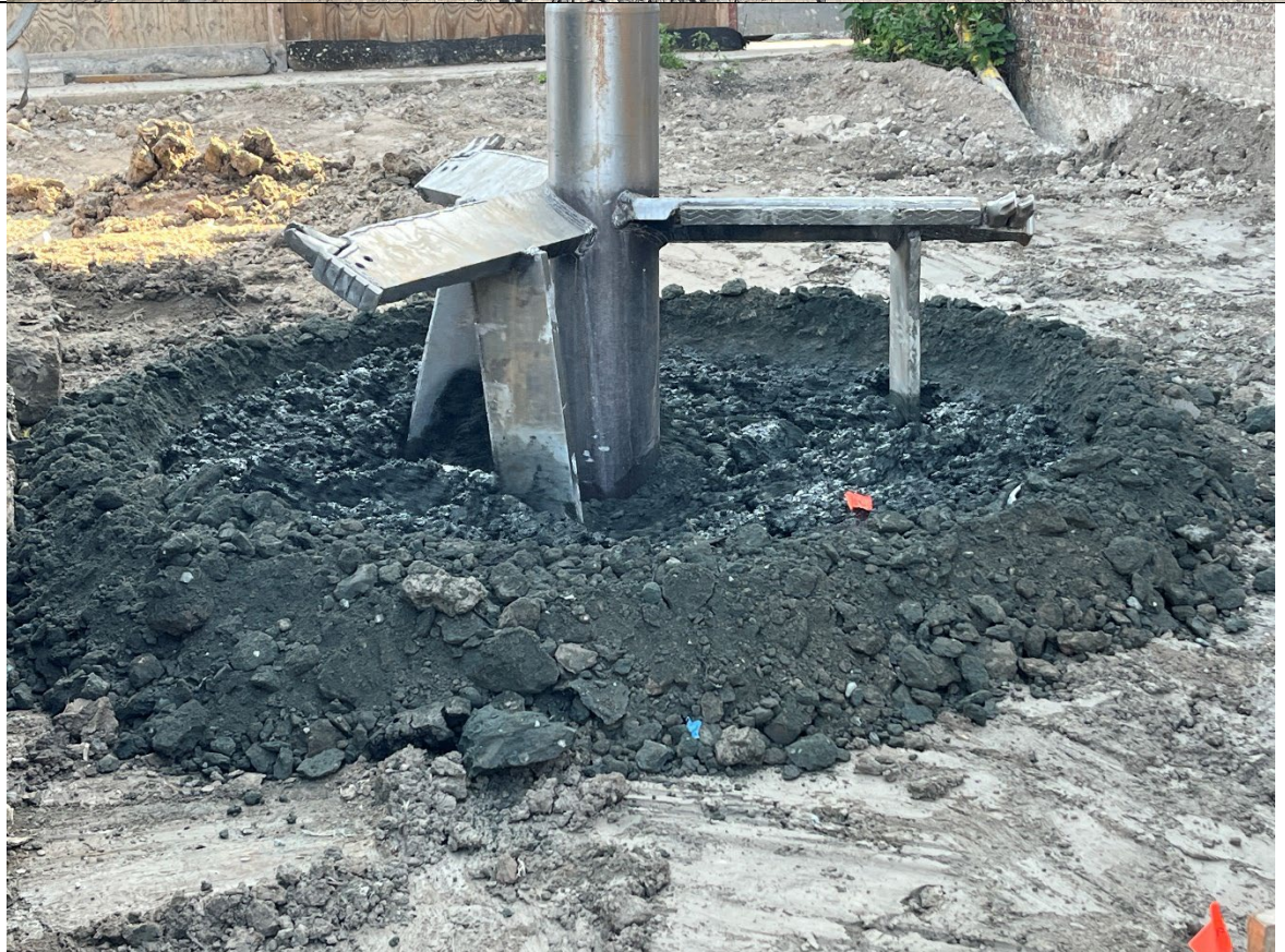
Photo 2- Representative photo of ISS Column installation.
