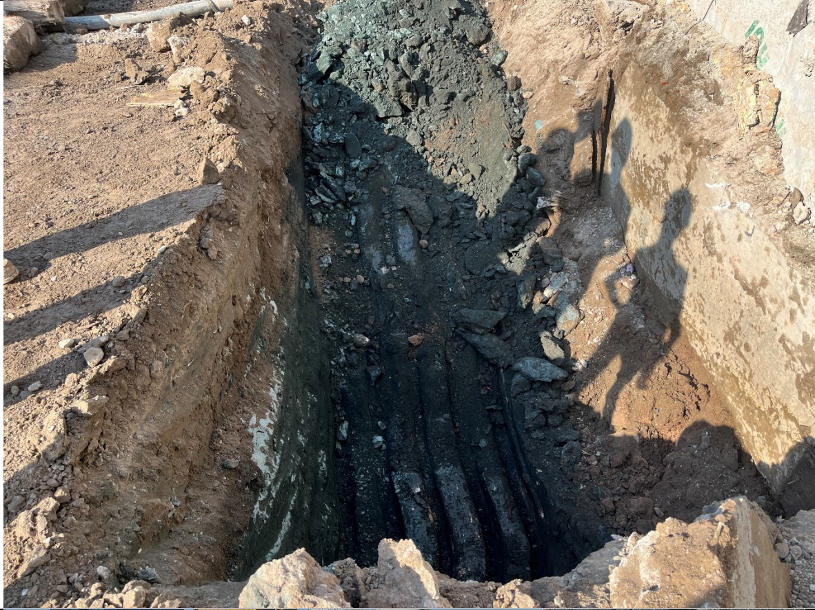
Photo 3- Representative photo of obstruction removal in southwestern portion of the alley.
