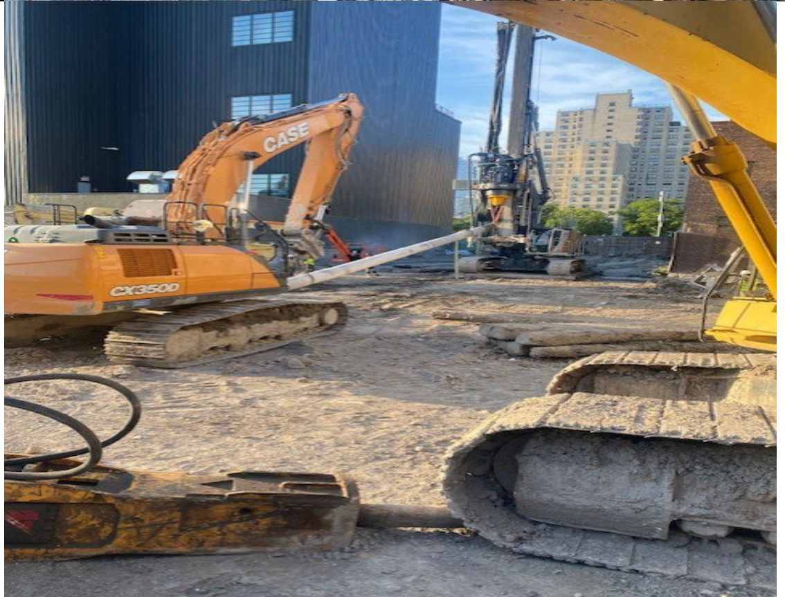
Photo 4- Representative photo of Cascade removing Kelly-bar from drill-rig.
