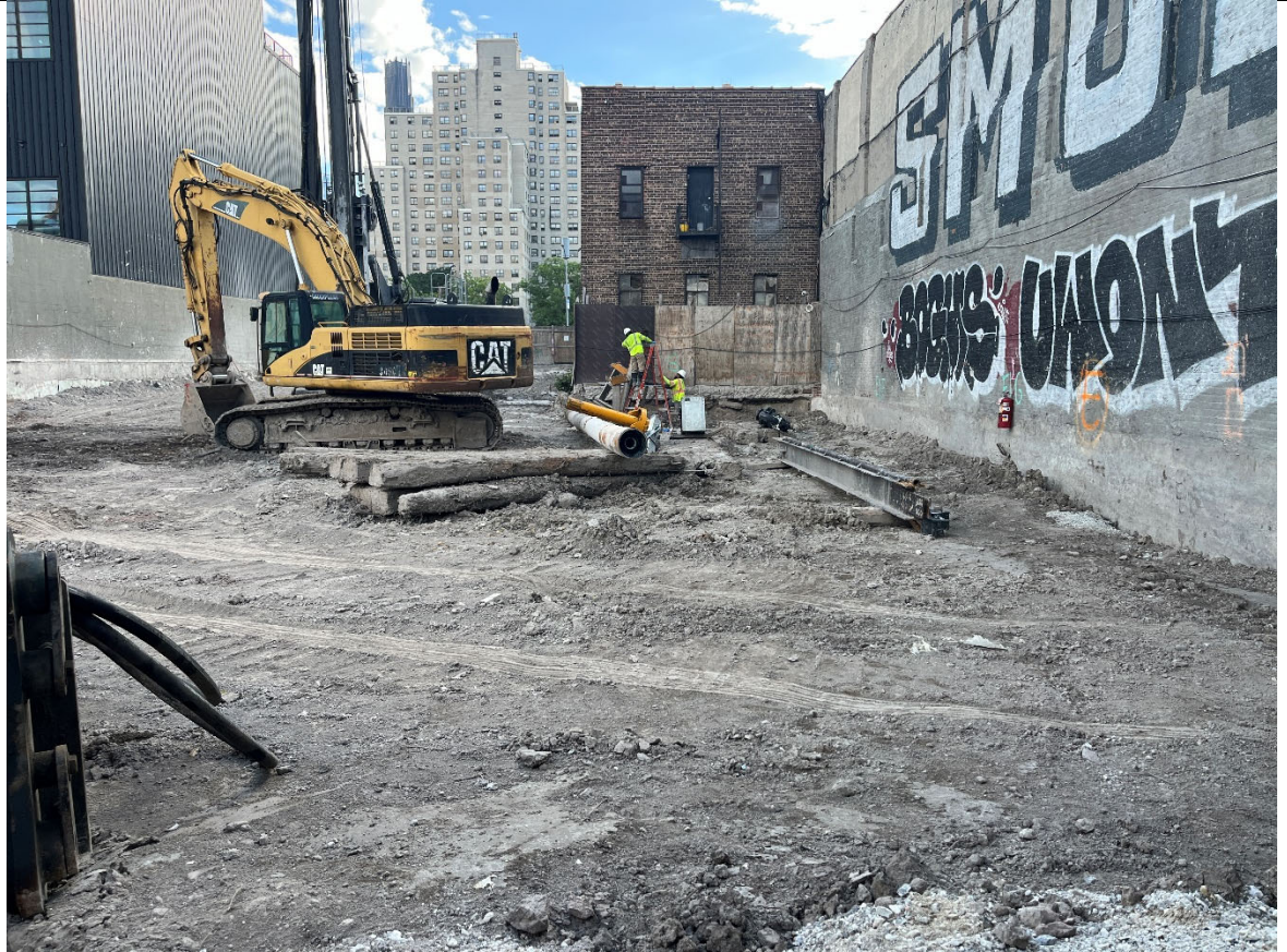
Photo 4- Representative photo of Cascade preparing Kelly bar and auger for assembly.
