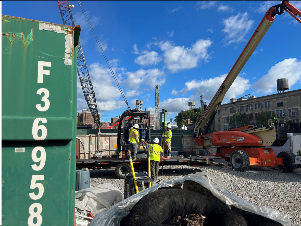
Photo 3- Representative photo of KDK delivery to the site.
