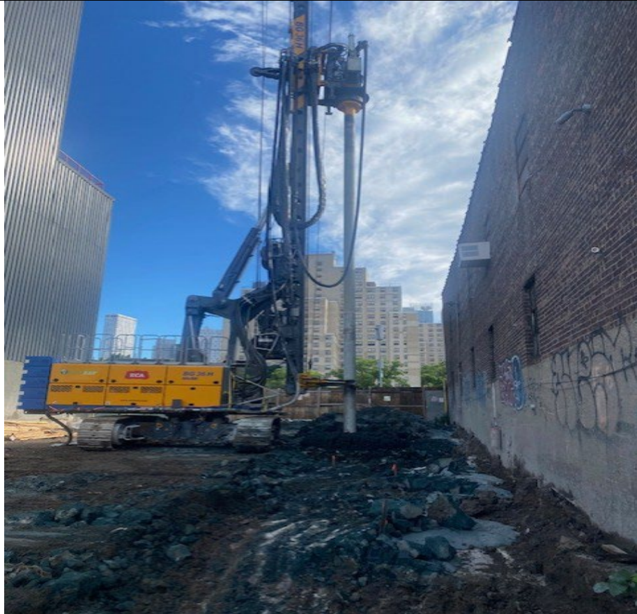
Photo 2- Representative photo of drill-rig installing ISS column.
