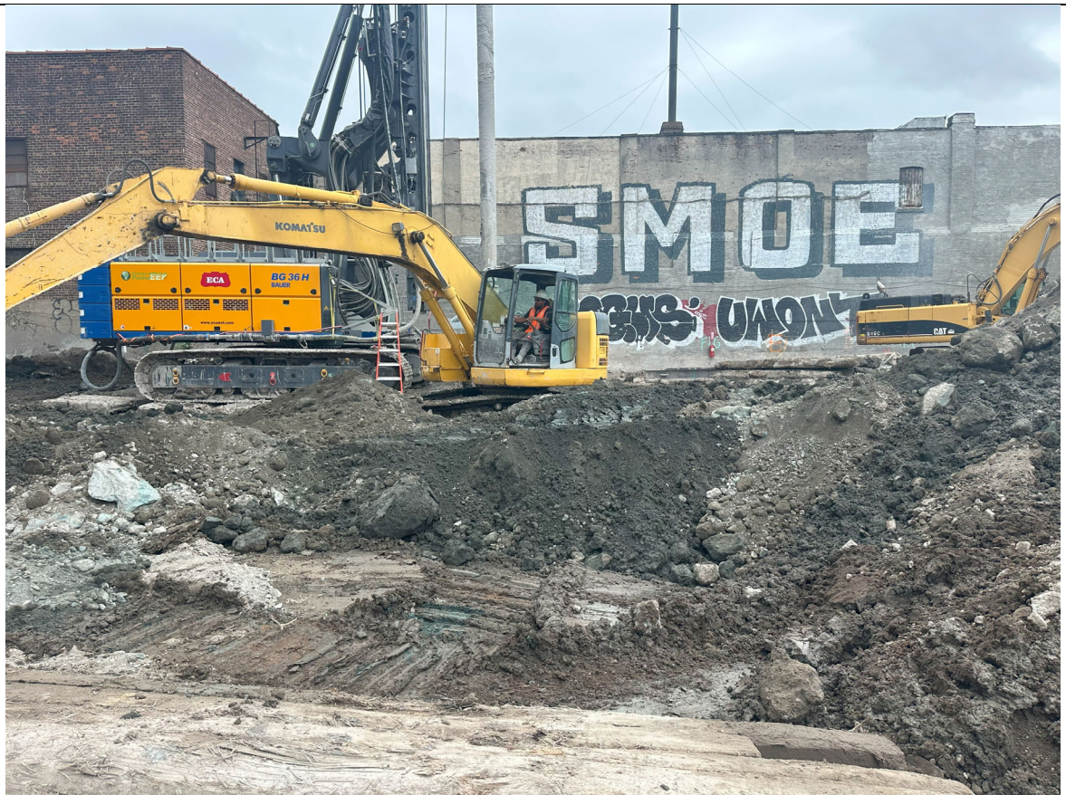
Photo 4- Representative photo of stock piling swell dirt.
