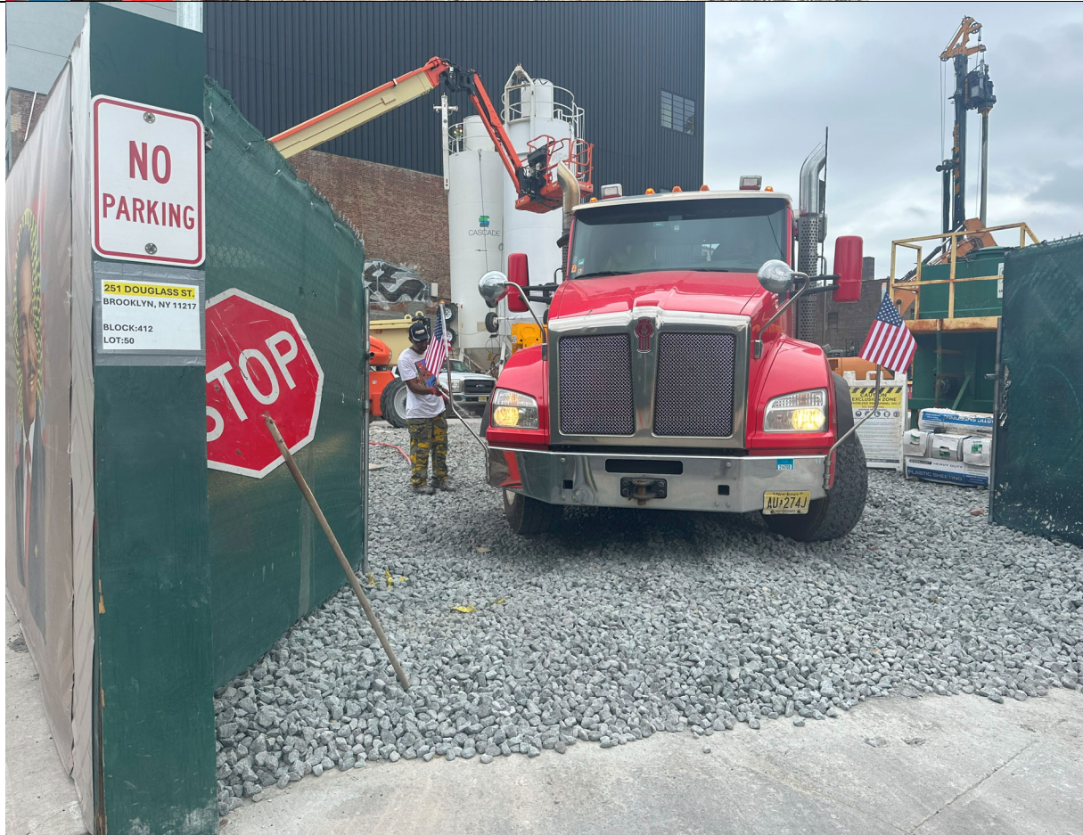
Photo 2- Representative photo of truck tires being washed off before exiting site.
