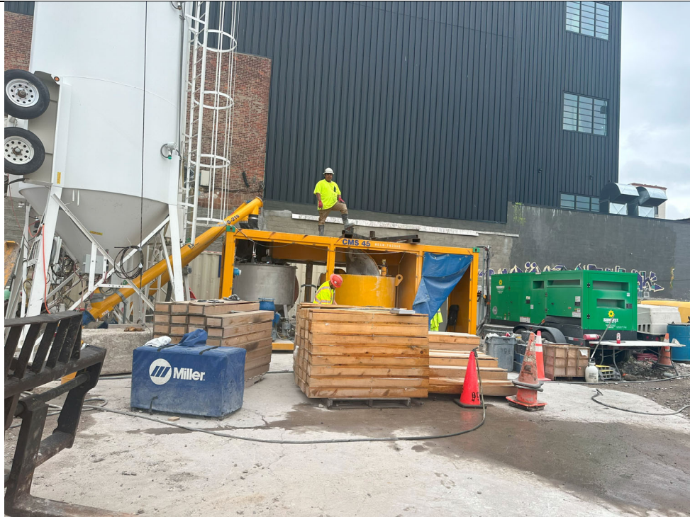
Photo 3- Representative photo of batch plant being maintained and serviced.
