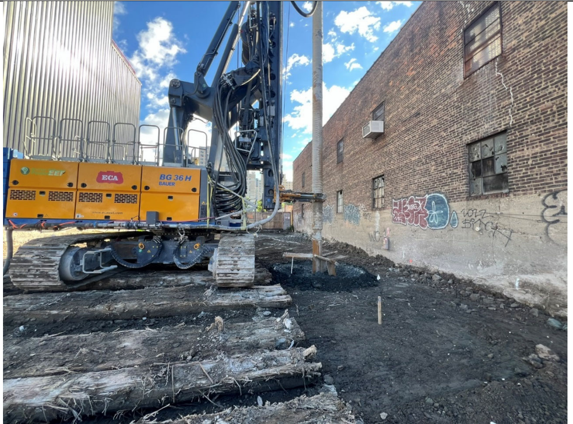
Photo 1- Representative photo of drilling an ISS column.
