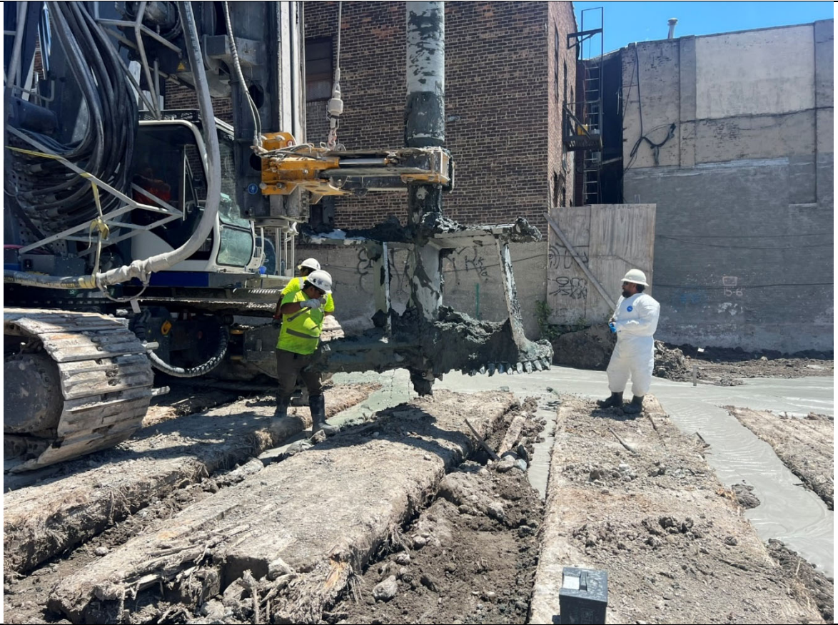
Photo 5- Representative photo of Cascade replacing teeth on the auger.
