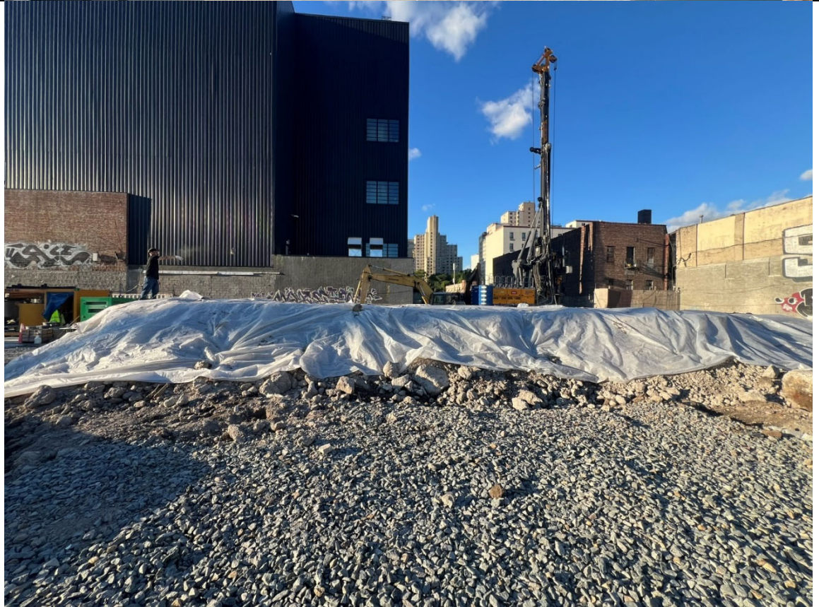
Photo 4- Representative photo of the swell stockpile covered at the end of the day.
