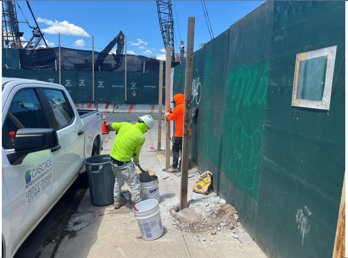
Photo 3- Representative photo of the fence being moved closer to the street.
