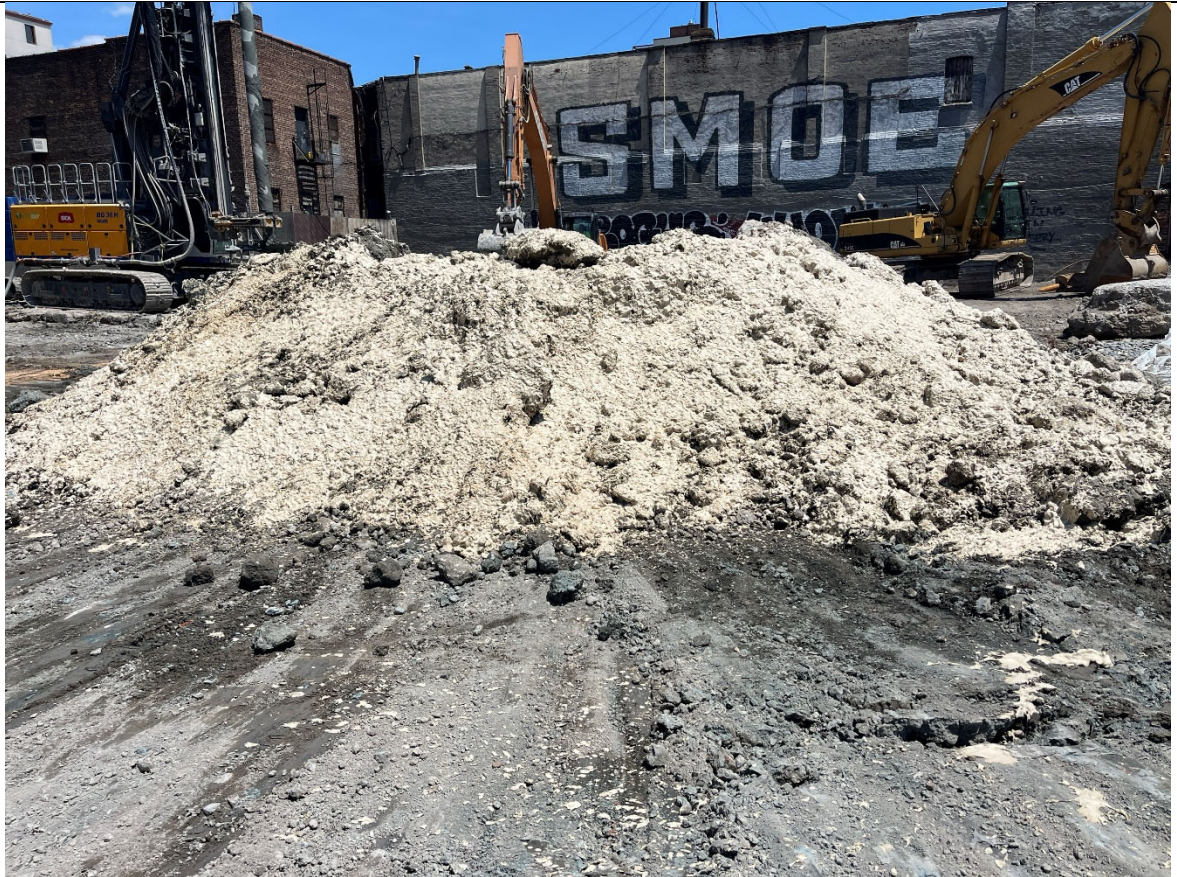
Photo 4- Representative photo of the swell stockpile covered in ATMOS foam when odors occurred during loadout.
