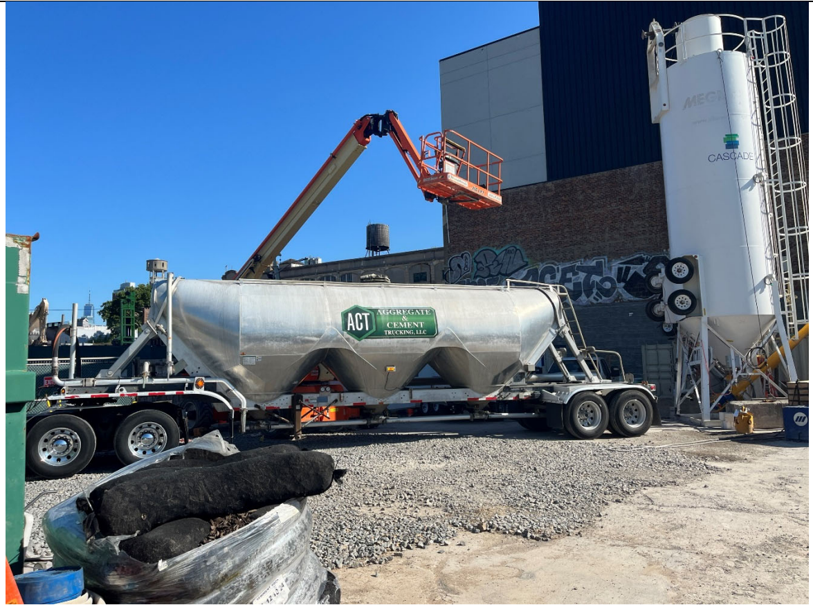
Photo 5- Representative photo of slag delivery.
