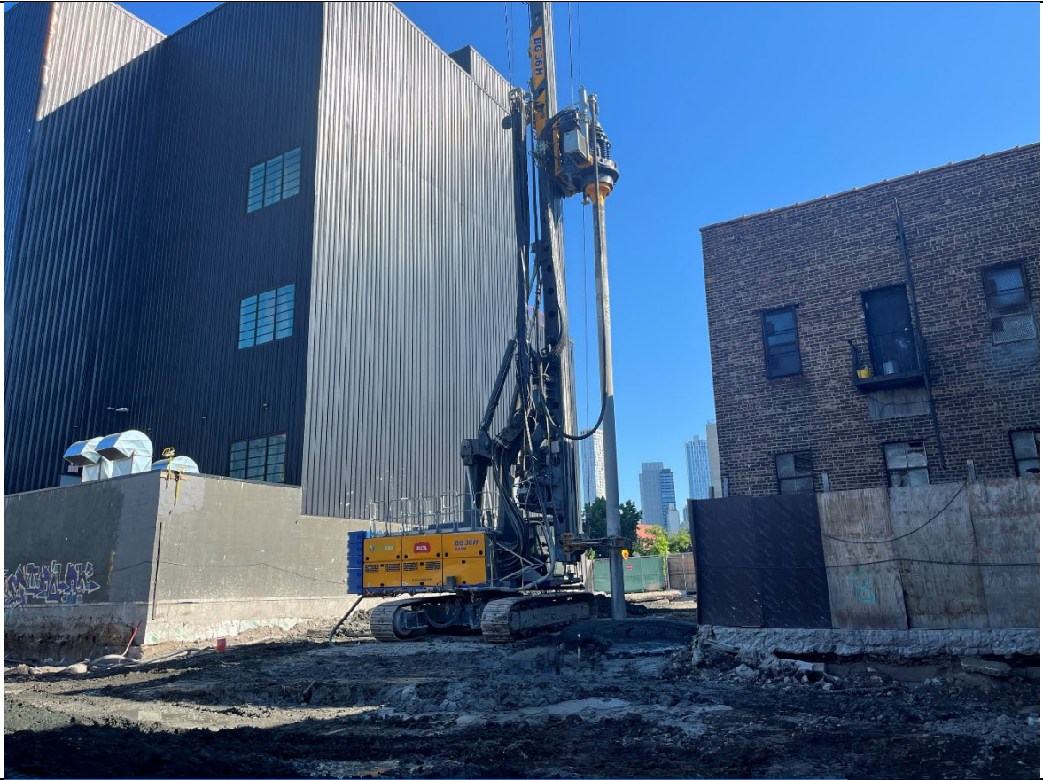
Photo 1- Representative photo of drilling an ISS column.
