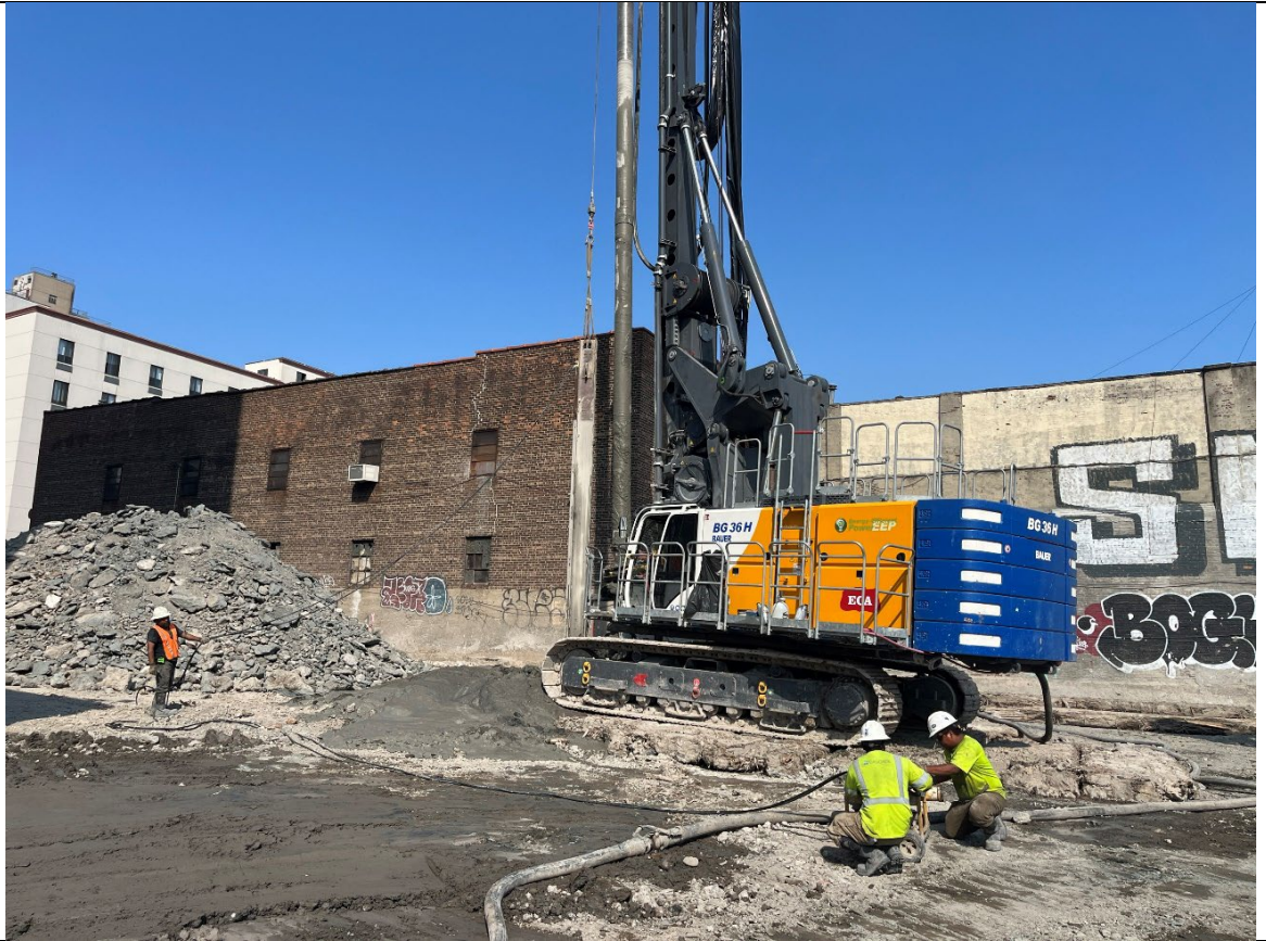
Photo 1- Representative photo of ISS wet mix sample collection from column 486.
