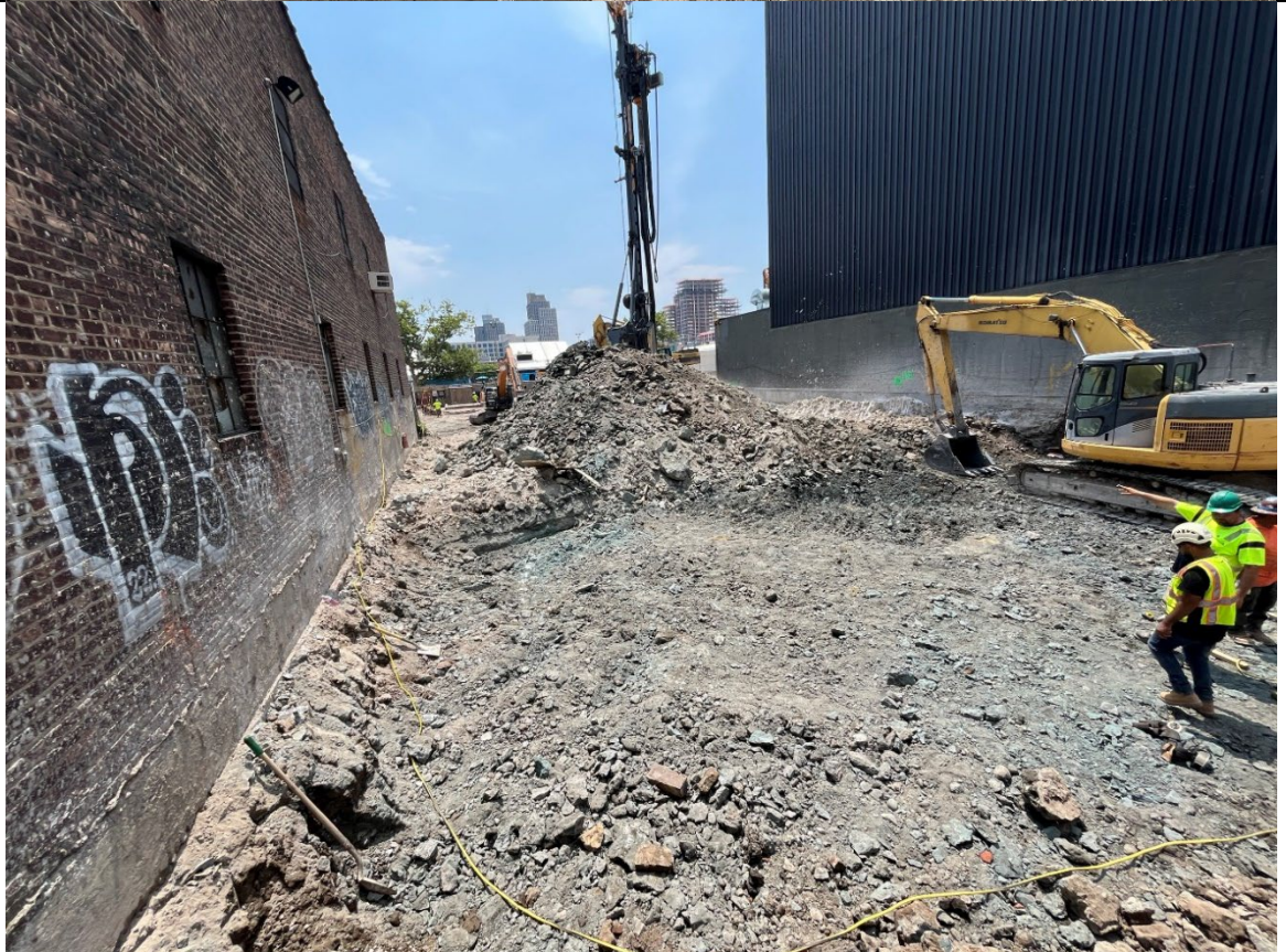
Photo 2- Representative photo of subgrade work in the Butler corridor.
