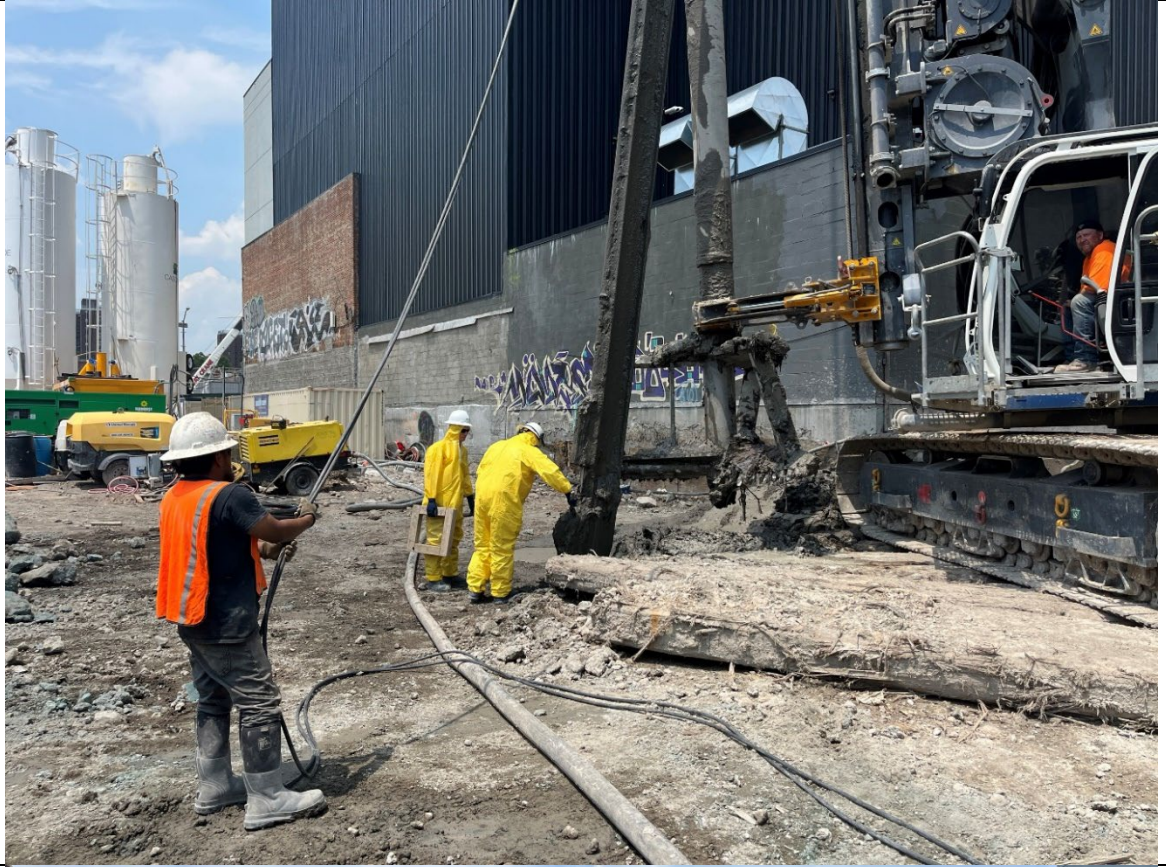
Photo 3- Representative photo of wet sample taken from Column 491.
