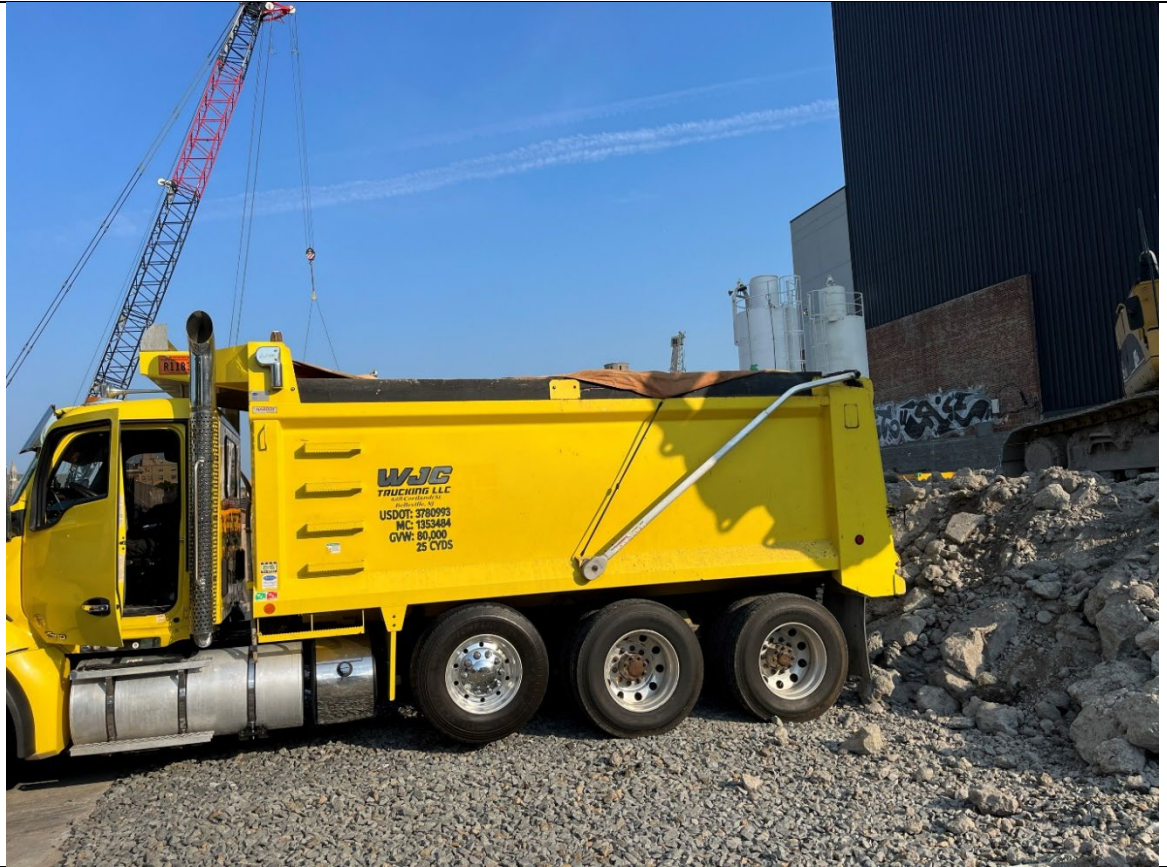
Photo 1- Representative photo of truck cover strapped down prior to exiting the Site.
