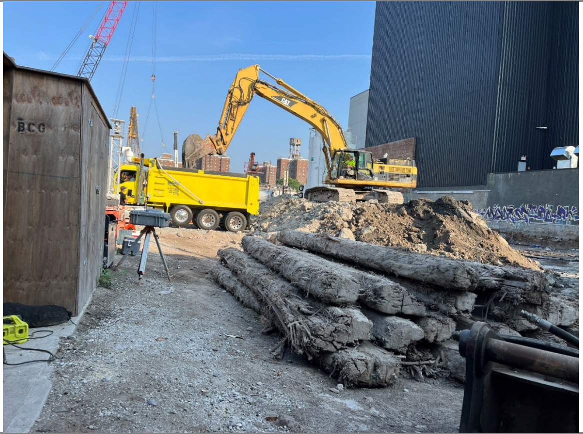
Photo 5- Representative photo of swell material loadout.
