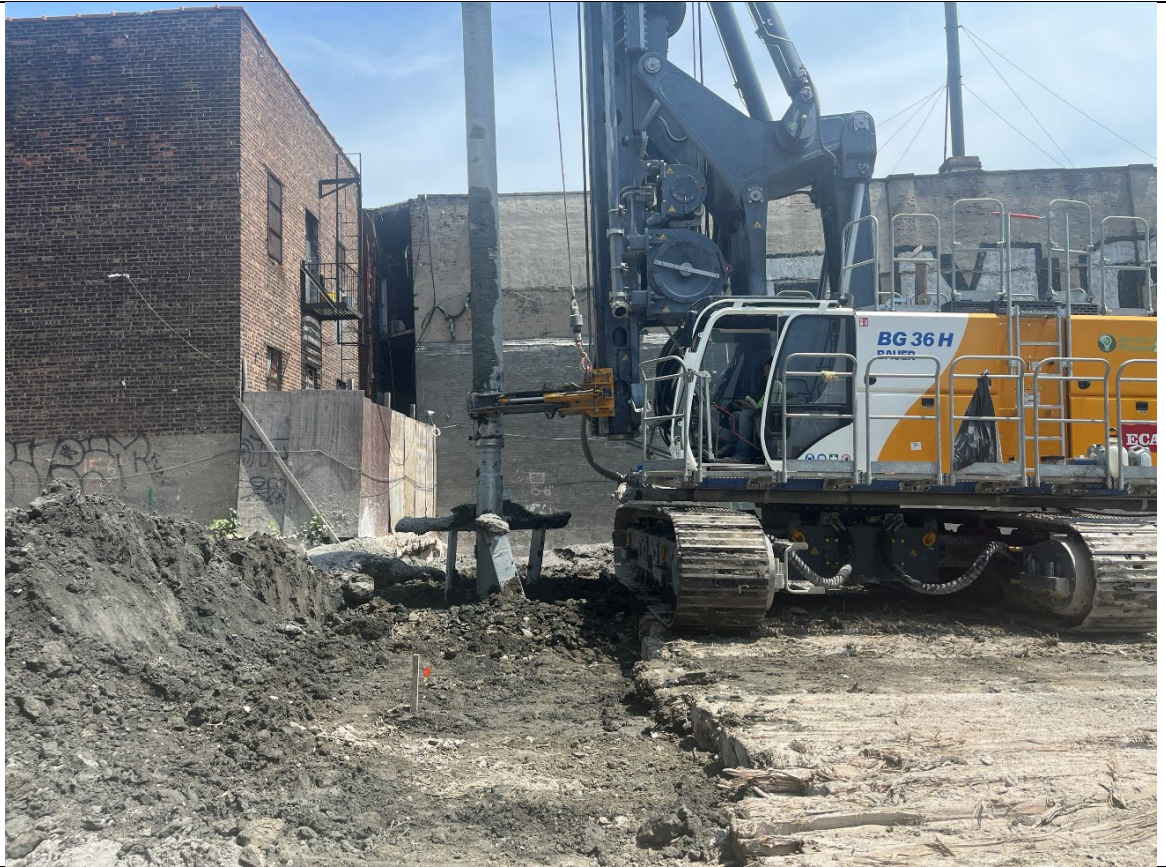
Photo 3- Representative photo of ISS column installation.
