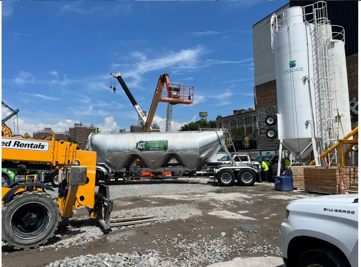
Photo 4- Representative photo of slag delivery to the silos.
