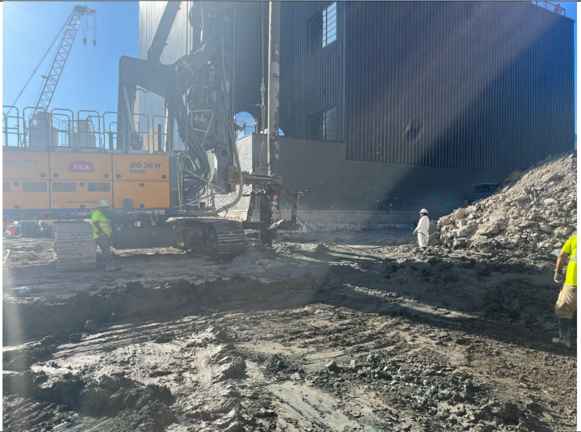
Photo 1- Representative photo of sampling rod collecting a wet mix sample from Column 472.
