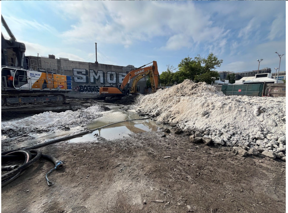
Photo 2- Representative photo of ATMOS foam sprayed on the swell stockpile.
