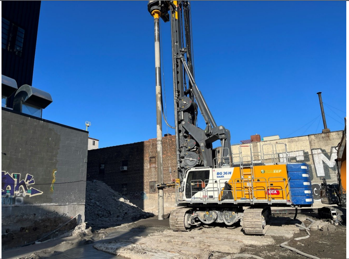
Photo 3- Representative photo of ISS column installation.
