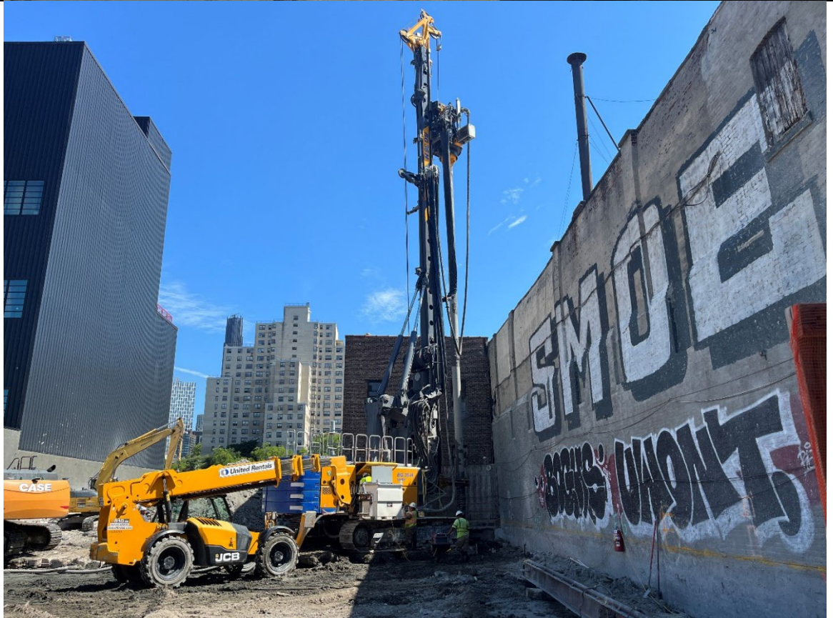
Photo 2- Representative photo of Cascade attempting to install column 480.
