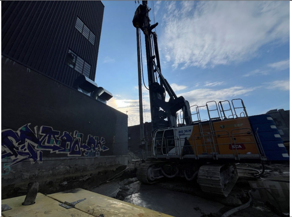
Photo 1- Representative photo of Column 492 installation.
