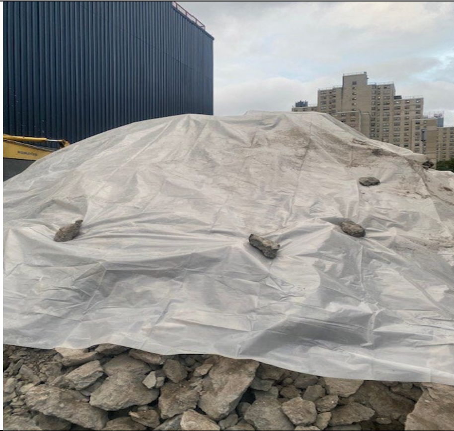
Photo 5- Representative photo of swell stockpile covered with poly- sheeting.
