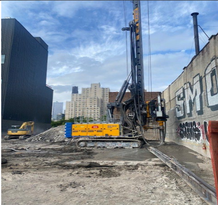
Photo 4- Representative photo of ISS column installation along eastern side of Site.
