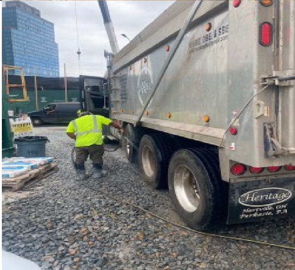
Photo 2- Representative photo of departing trucks passing through wash-station prior to exiting the Site.
