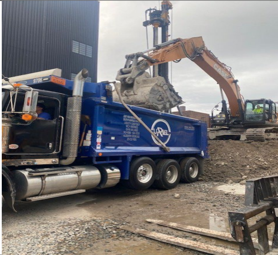
Photo 1- Representative photo of swell load-out for disposal at Bayshore.
