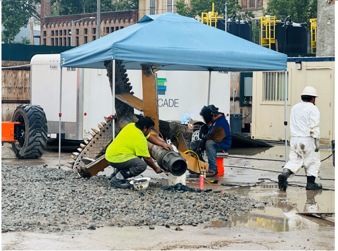
Photo 3- Representative photo of rig auger being welded and serviced.
