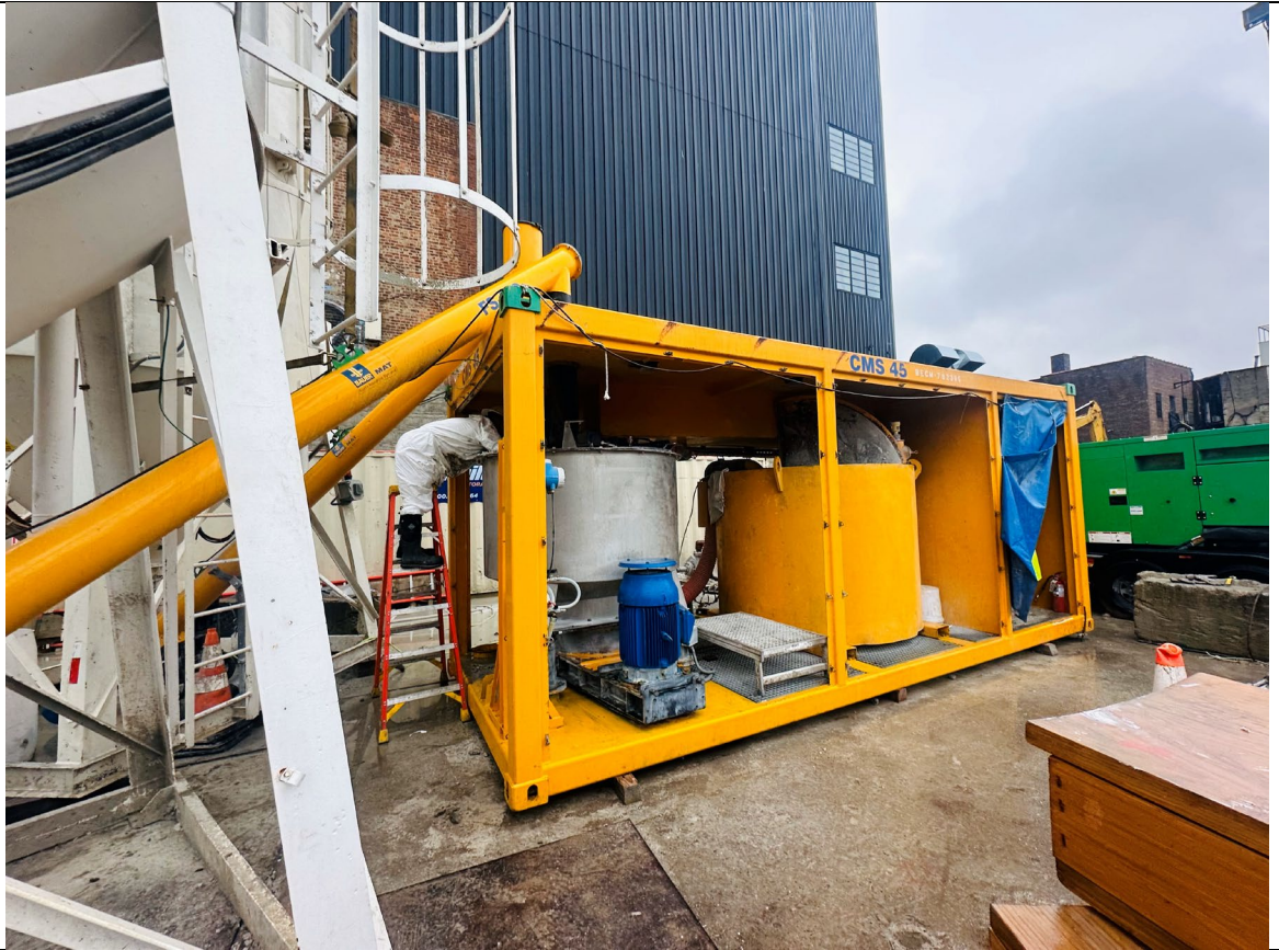
Photo 1- Representative photo of batch plant being cleaned out and serviced.
