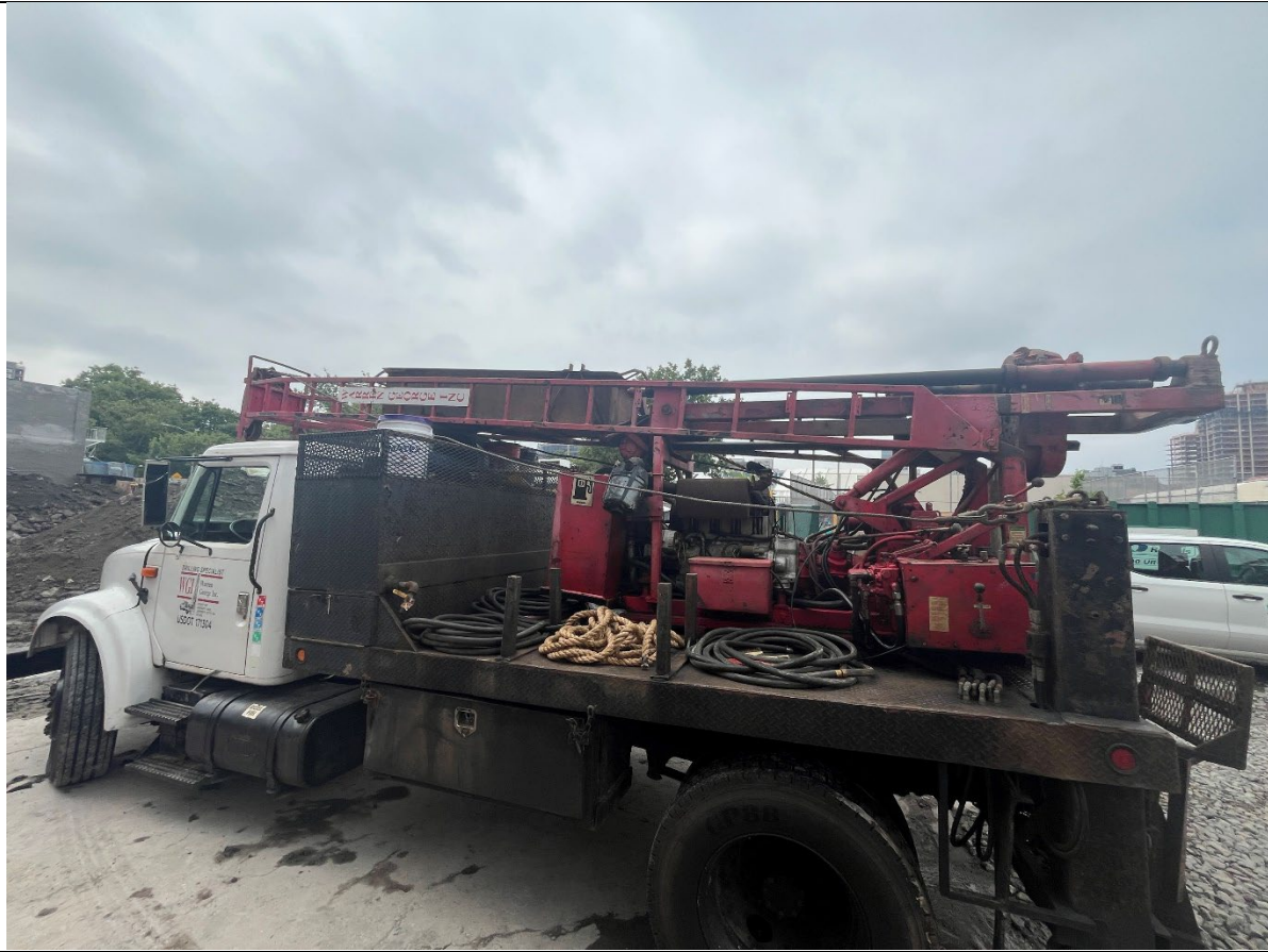
Photo 5- Representative photo of WGI bringing coring equipment onsite.
