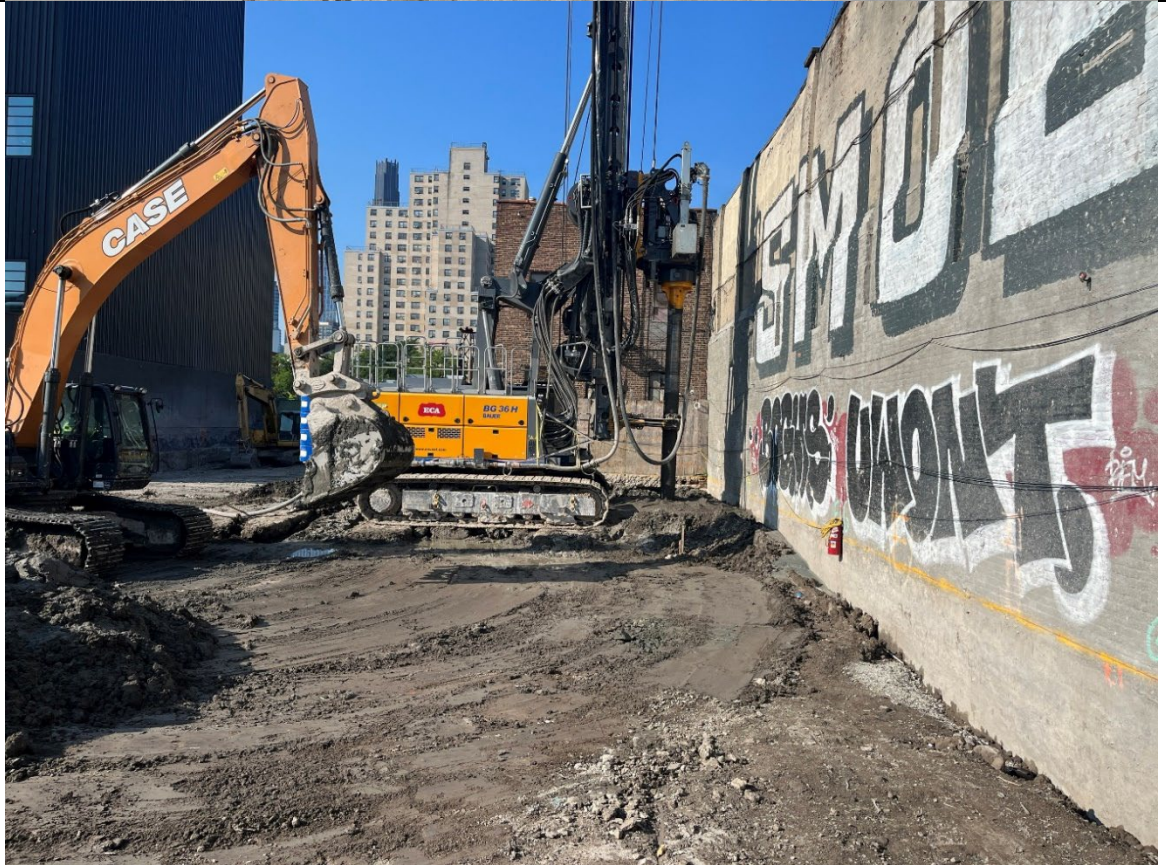
Photo 4- Representative photo of ISS column installation along eastern side of Site.
