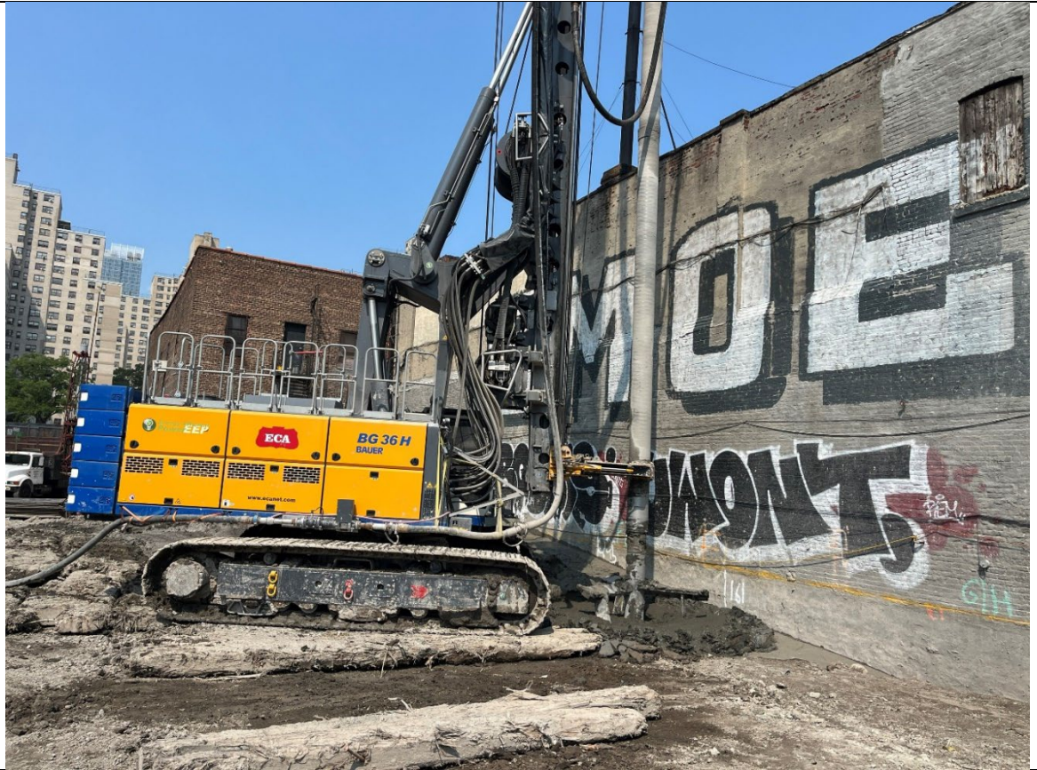
Photo 1- Representative photo of ISS column installation.
