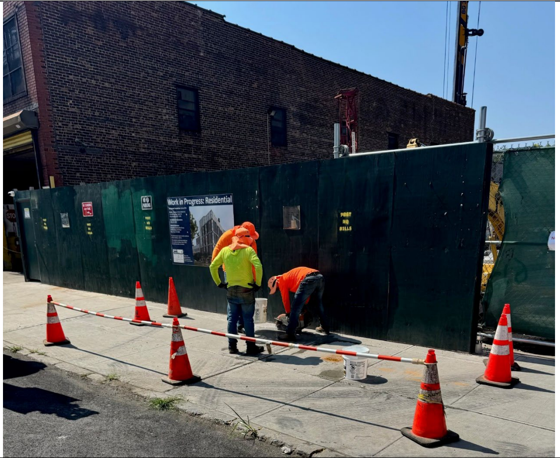
Photo 5- Representative photo of Empire beginning sidewalk work.
