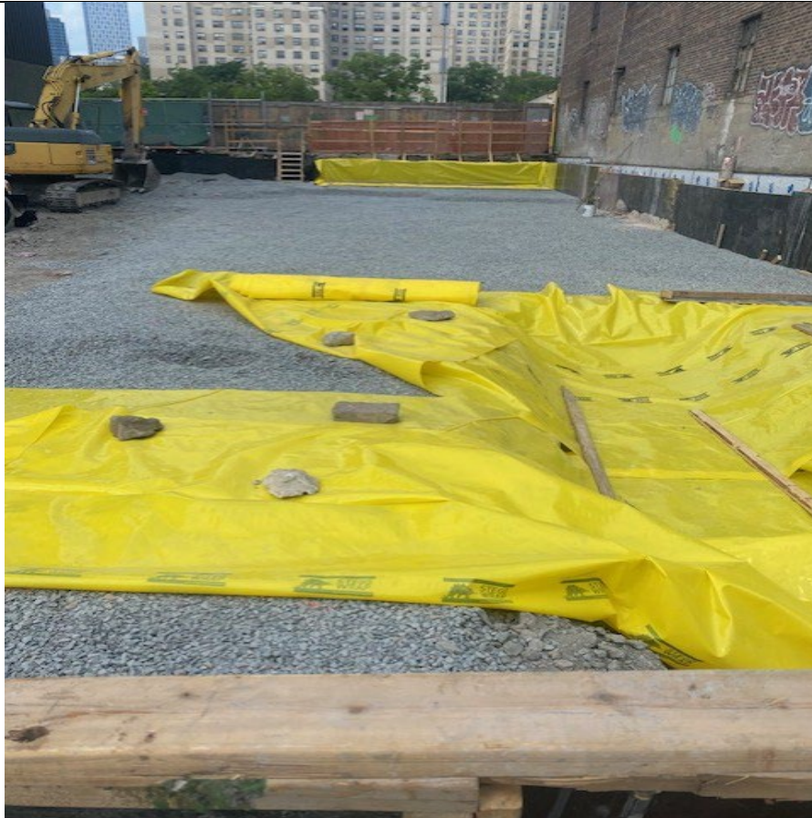
Photo 3- Representative photo of sub- grade work along northern alley.
