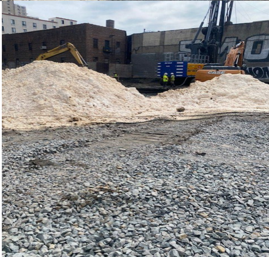
Photo 2- Representative photo of swell material stockpile covered with Atmos foam odor suppressant.
