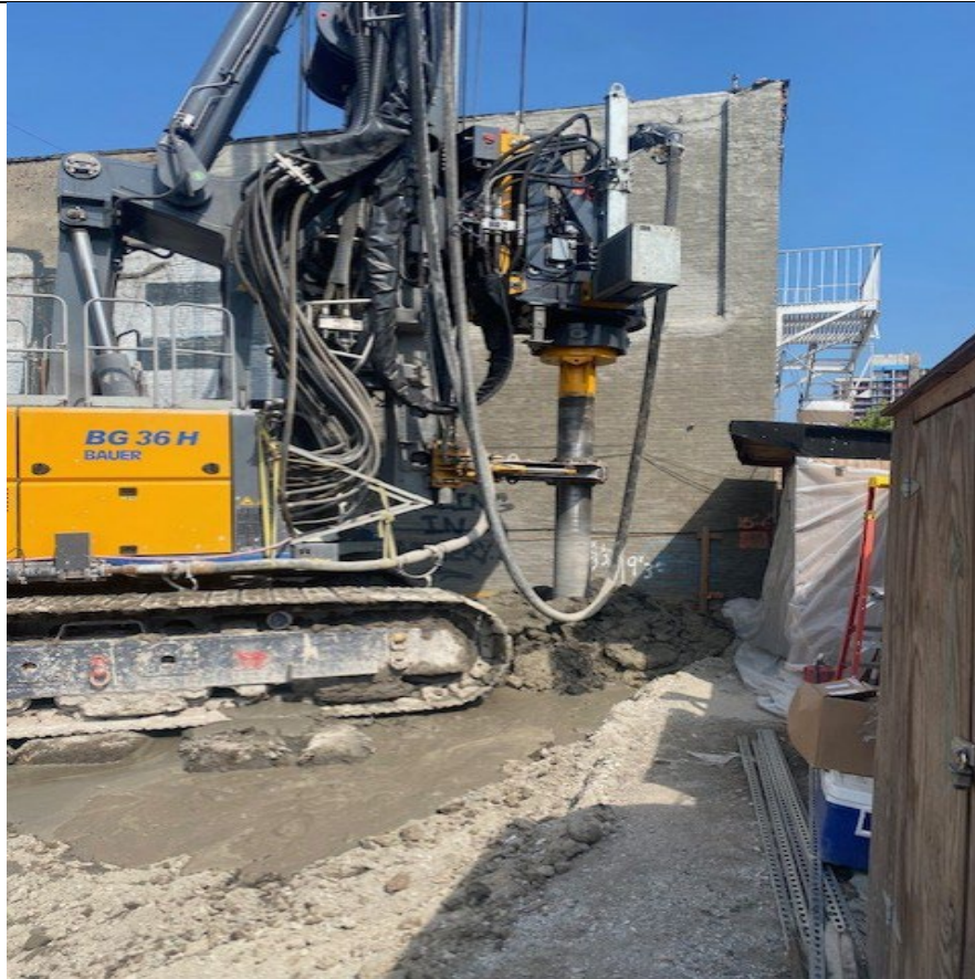
Photo 1- Representative photo of ISS column installation at southeastern corner of property.
