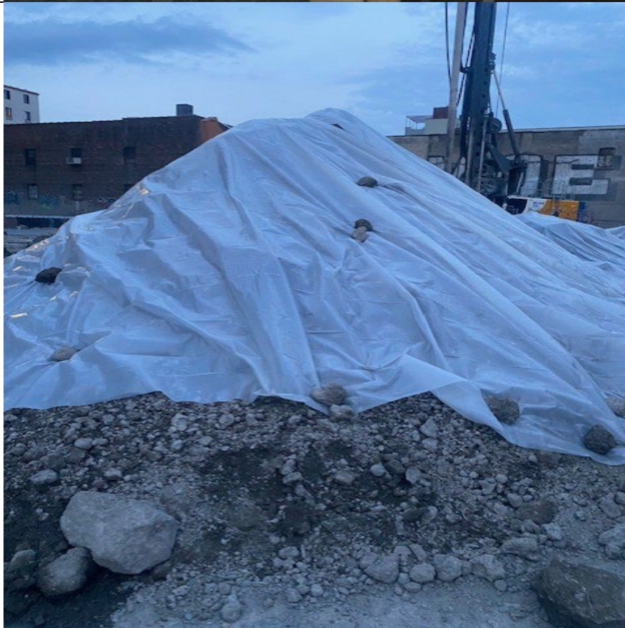
Photo 4- Representative photo of swell stockpile covered with poly- sheeting.
