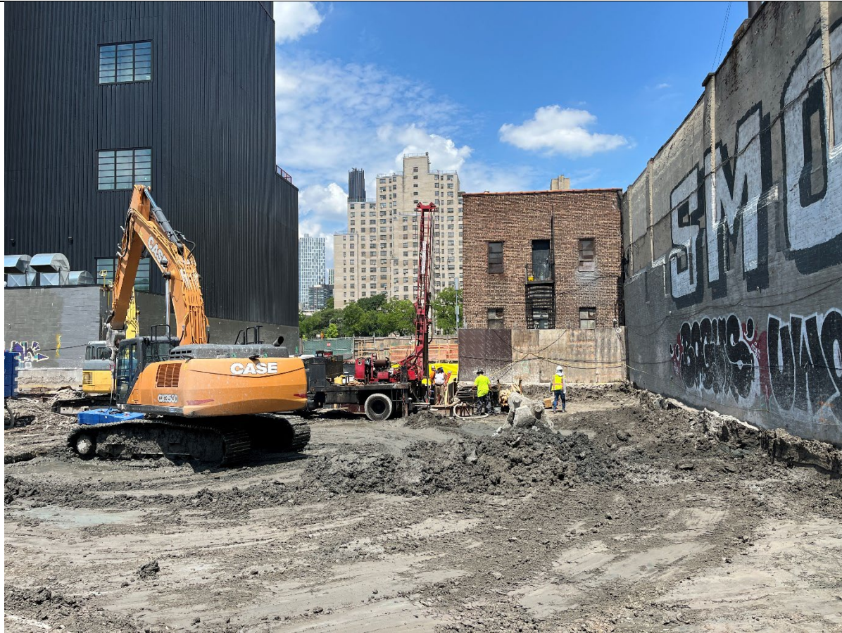
Photo 5- Representative photo of structural stability coring performed by WGI and GES.
