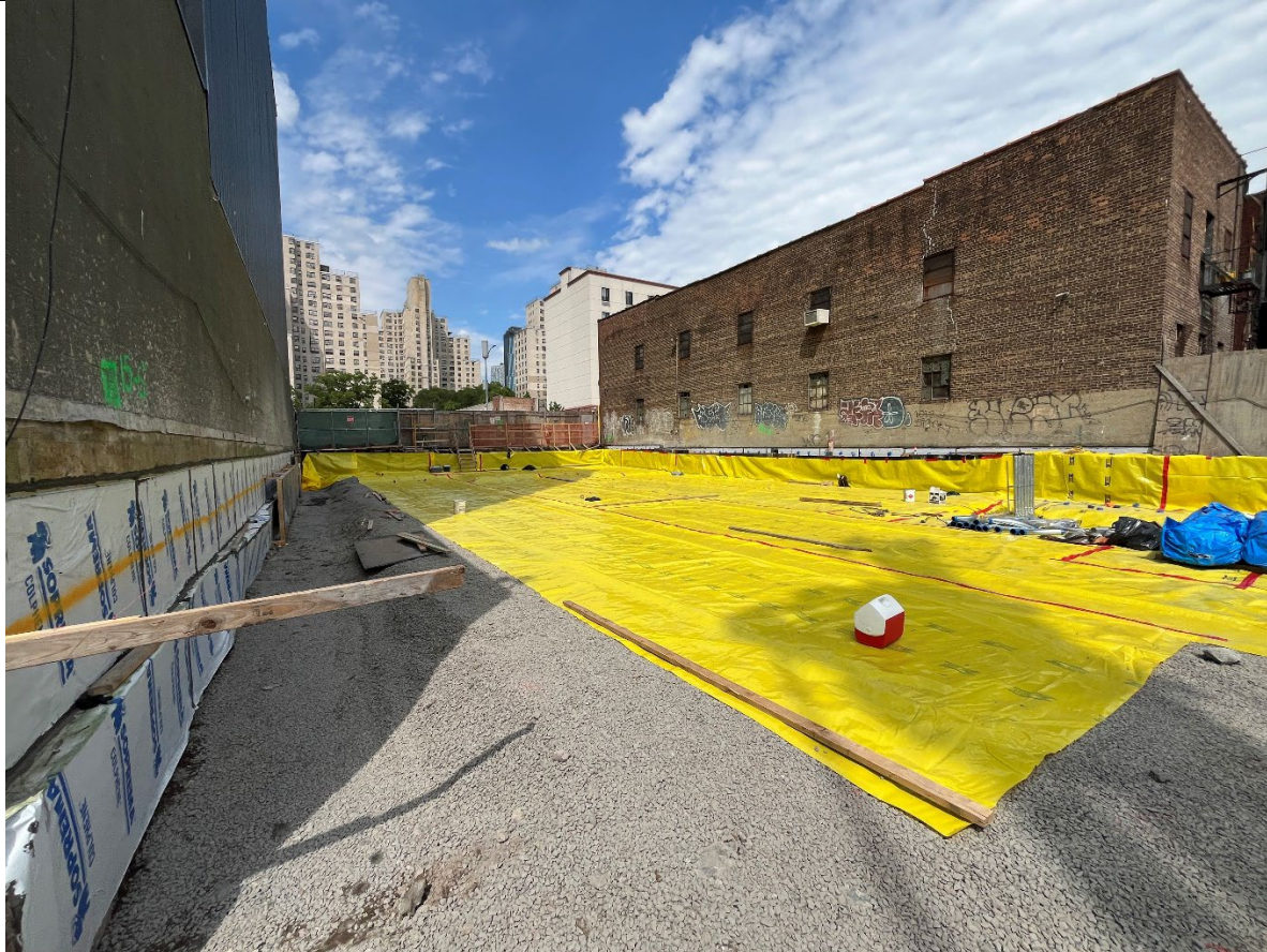
Photo 2- Representative photo of vapor barrier installed in the Butler Corridor.
