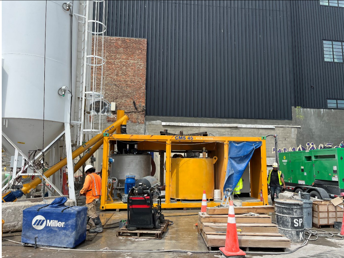
Photo 4- Representative photo of Cascade cleaning the ISS batch plant.
