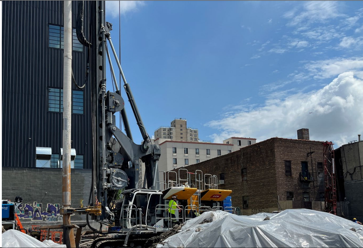
Photo 3- Representative photo of ECA servicing the ISS drill rig.
