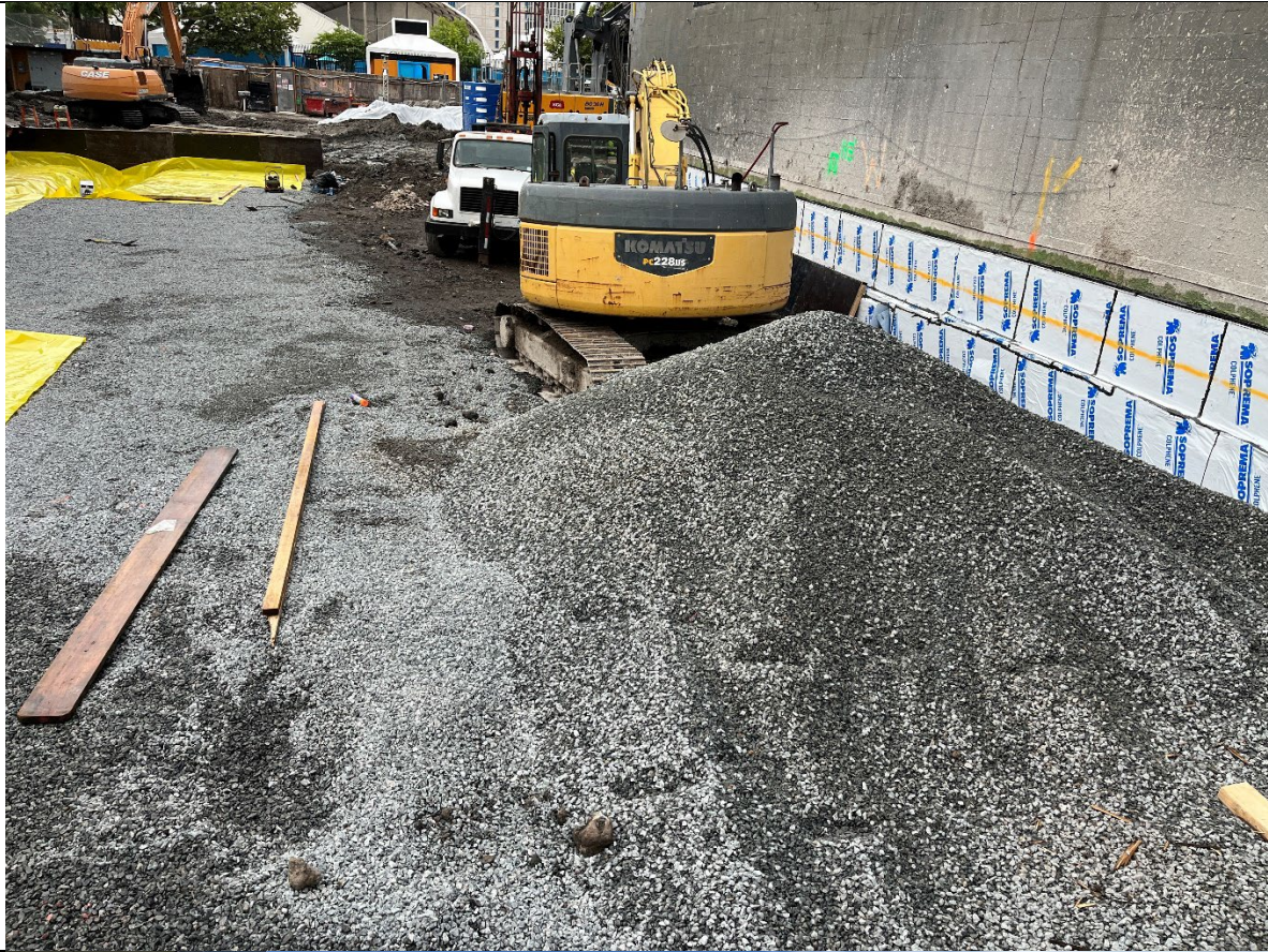
Photo 1- Representative photo of approved 3/4" stone delivered to the Butler Corridor.
