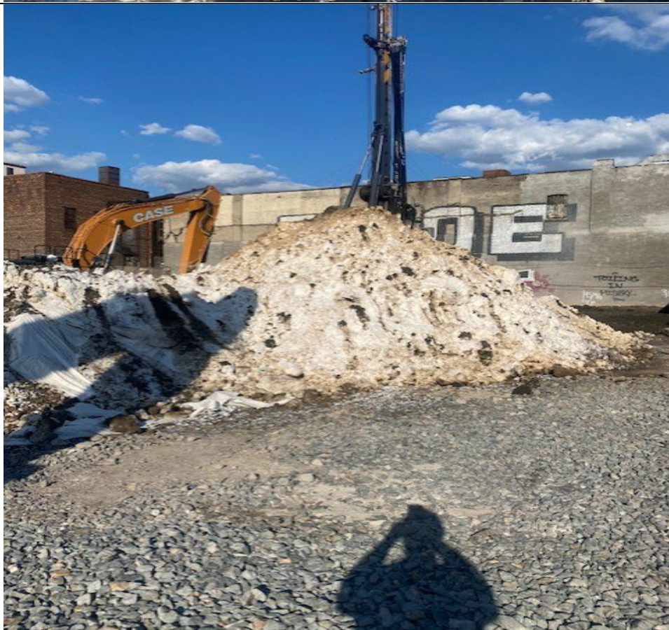
Photo 4- Representative photo of swell material stockpile covered with Atmos foam odor suppressant.
