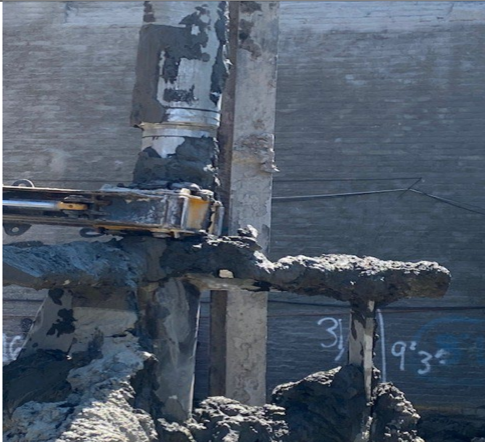
Photo 3- Representative photo of wet- sample collected from completed ISS column by use of bar.
