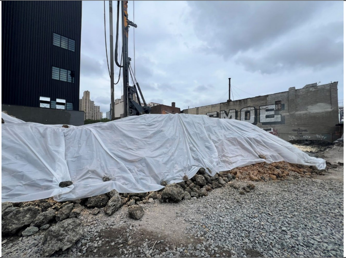
Photo 5- Representative photo of the swell stockpile covered at the end of the day.
