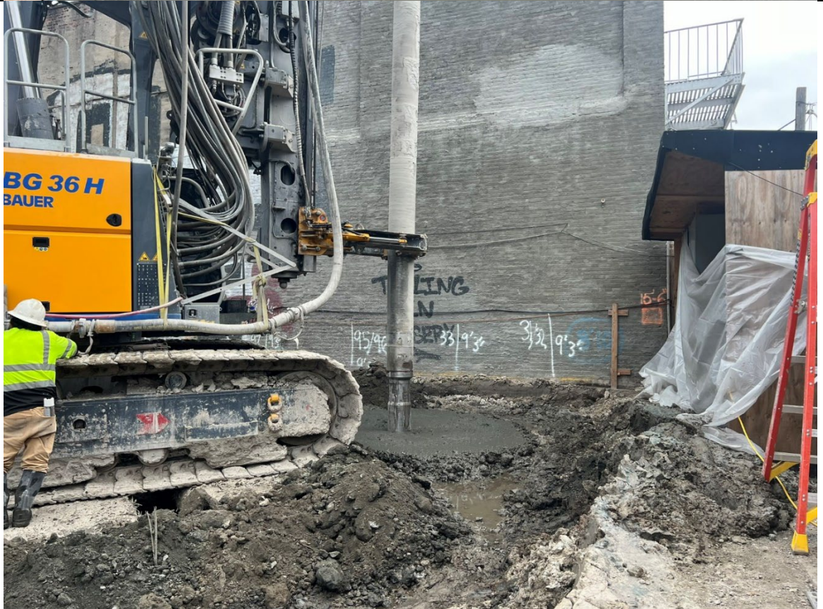
Photo 4- Representative photo of drilling an ISS Column.
