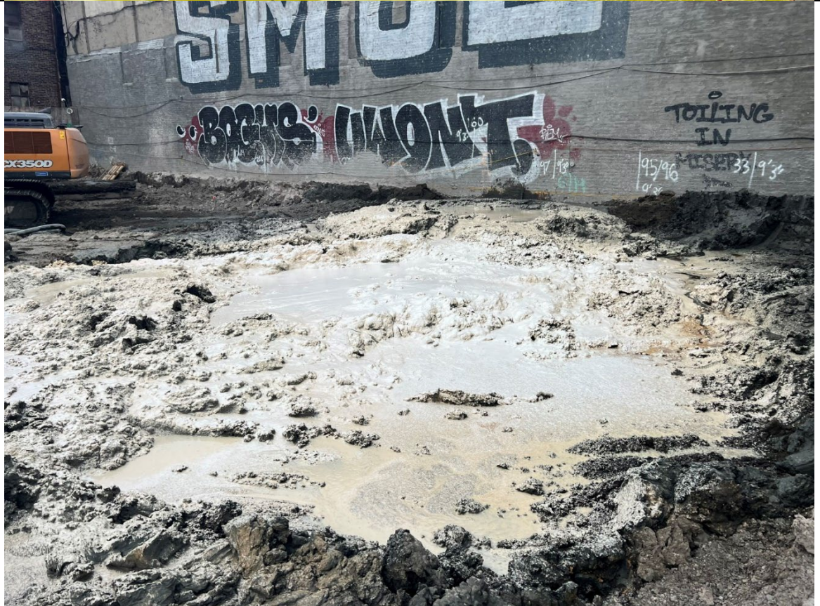
Photo 2- Representative photo of the work area sprayed with Atmos Foam.
