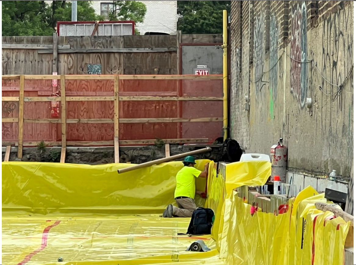
Photo 1- Representative photo of Concrete Courses fixing the vapor barrier.
