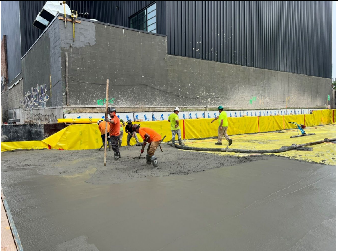
Photo 3- Representative photo of the mat slab being poured.
