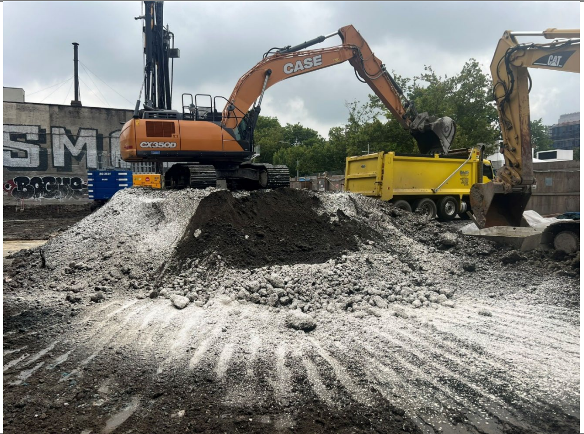
Photo 3- Representative photo of swell material being removed for offsite disposal.
