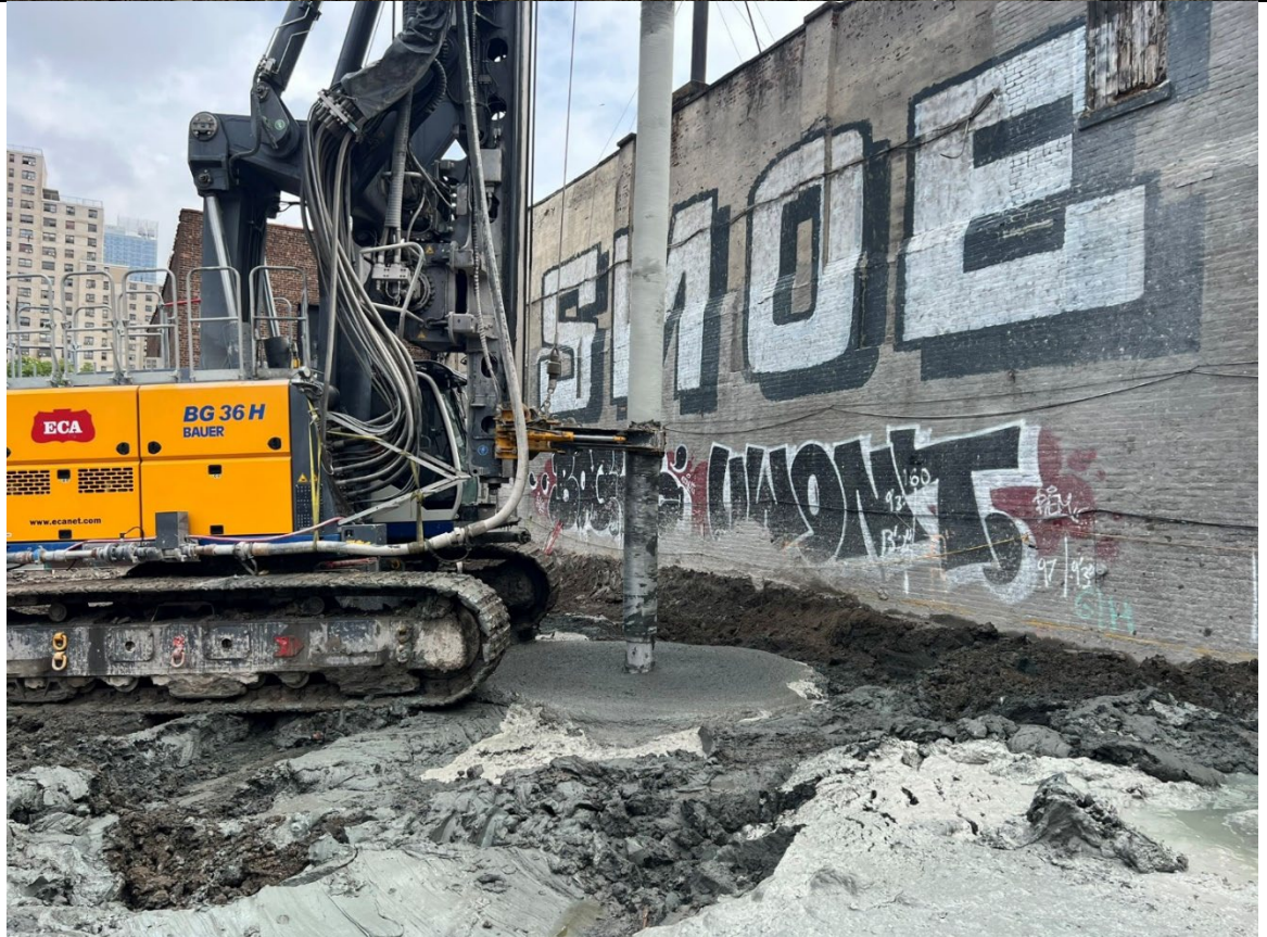
Photo 4- Representative photo of drilling an ISS Column.
