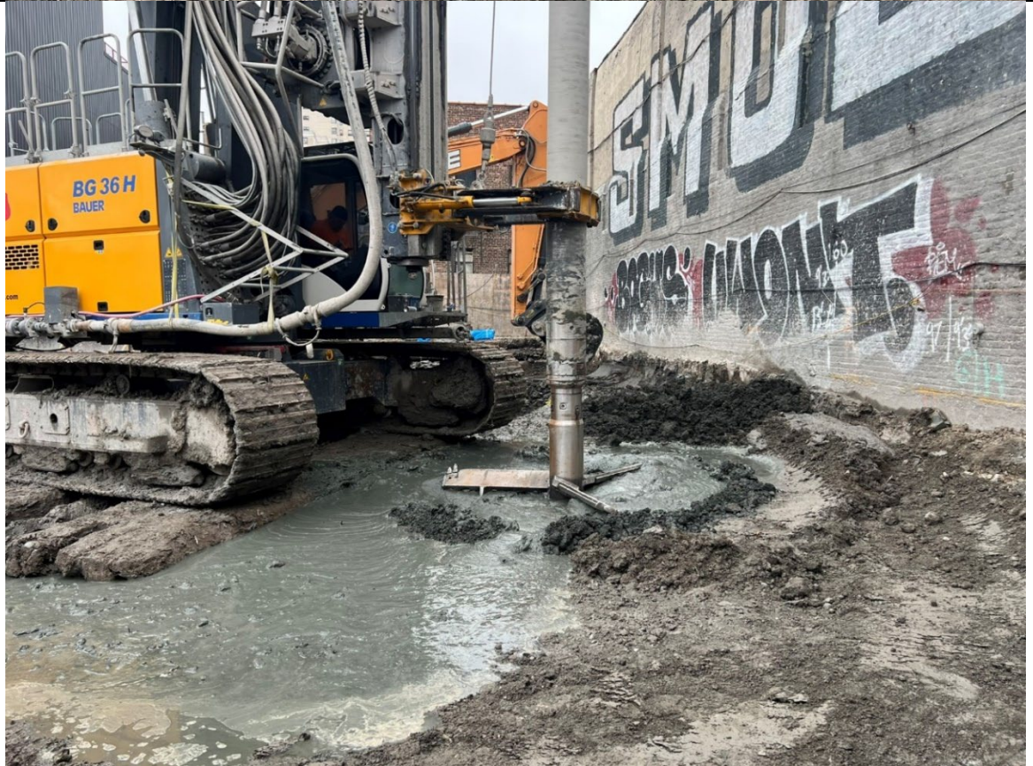
Photo 4- Representative photo of drilling an ISS Column.
