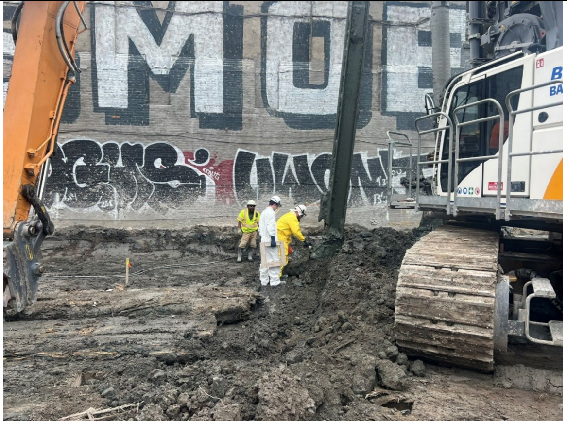
Photo 3- Representative photo of a wet mix sample being collected from Column 98 at 32'.
