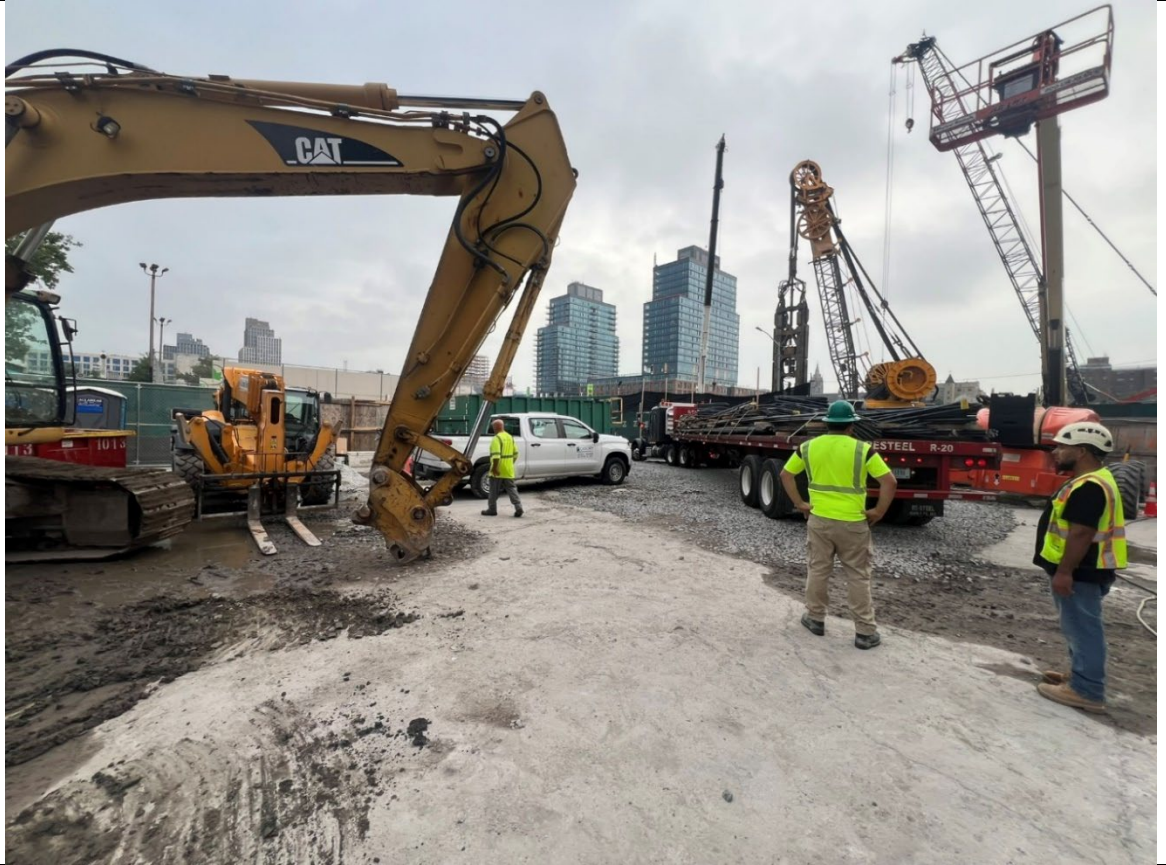
Photo 1- Representative photo of rebar being delivered.
