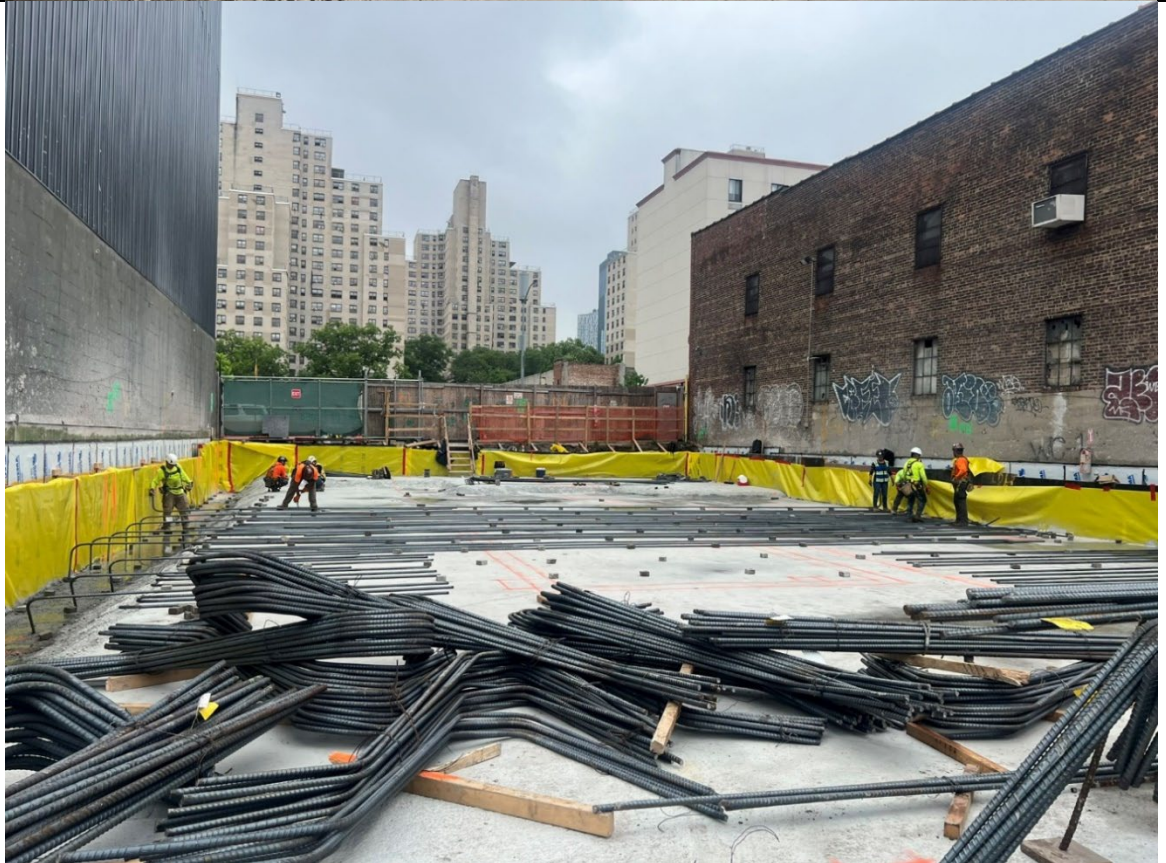
Photo 2- Representative photo of Concrete Courses laying rebar.
