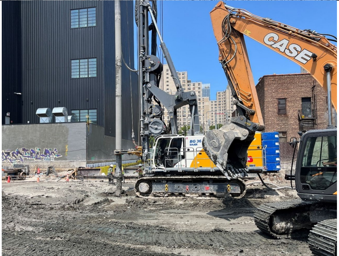
Photo 4- Representative photo of drilling an ISS Column.
