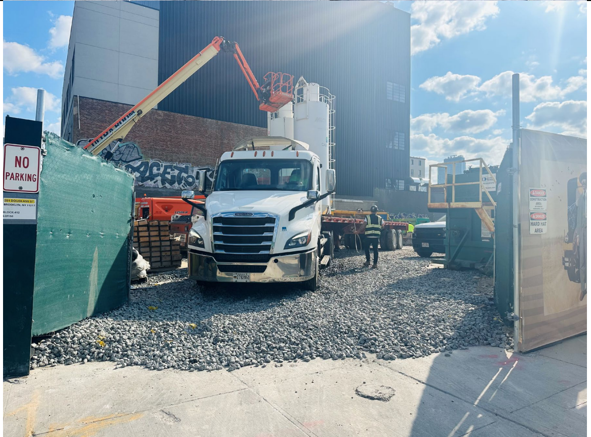
Photo 2- Representative photo of delivery truck tires being washed before exiting site.
