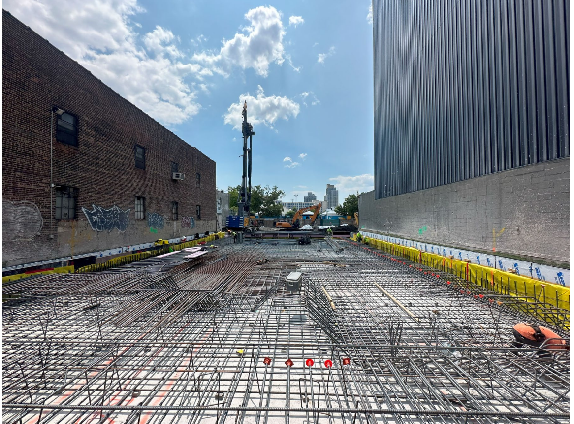
Photo 4- Representative photo of rebar installation by Concrete Course.
