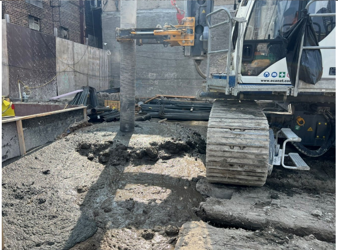
Photo 2- Representative photo of an ISS column being drilled.
