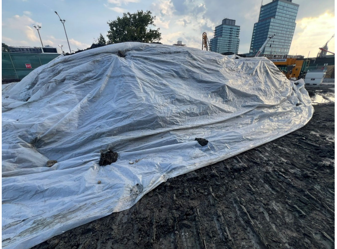
Photo 4- Representative photo the ISS swell pile covered the end of the day.
