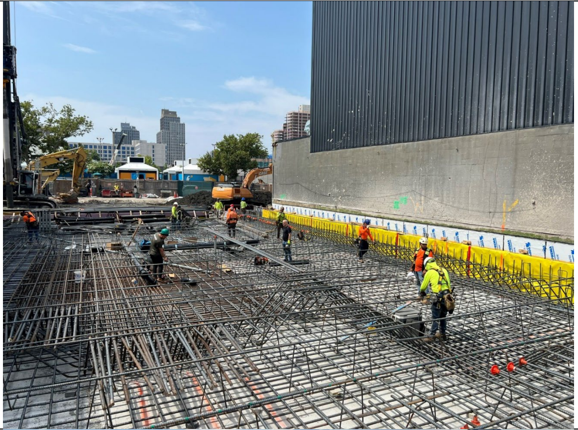
Photo 3- Representative photo of rebar work in the Butler corridor.
