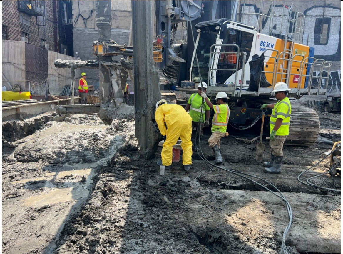
Photo 2- Representative photo of wet mix sample collection at Column 421 at 29' bgs.
