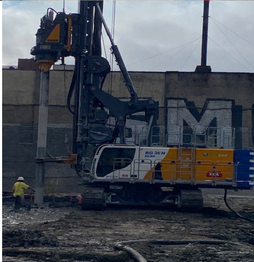
Photo 2- Representative photo of an ISS column being drilled.
