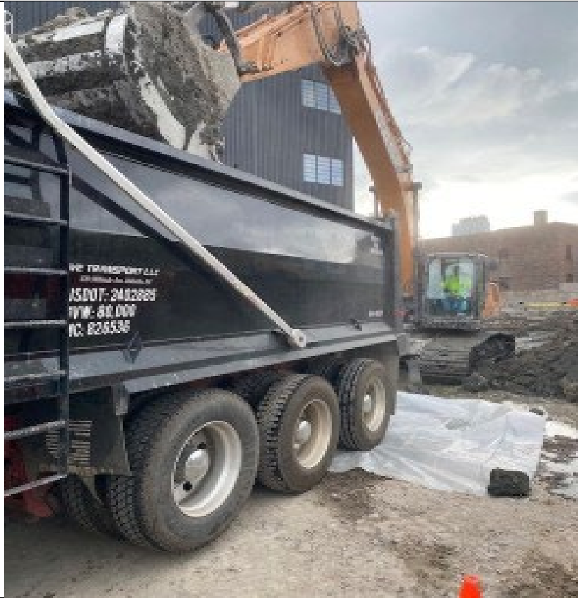
Photo 1- Representative photo of swell material loading atop poly-sheeting.
