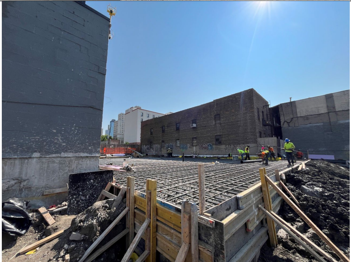
Photo 2- Representative photo of rebar work in the Butler corridor.
