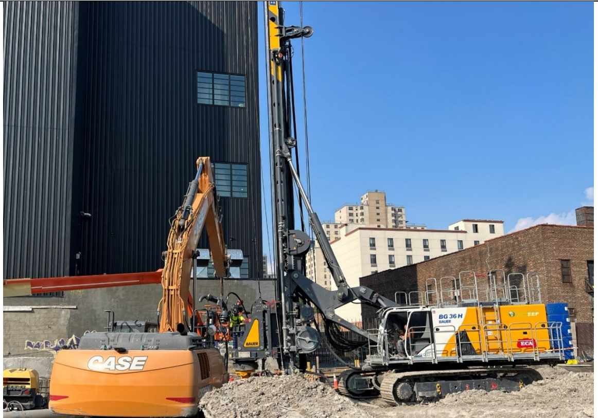
Photo 1- Representative photo of installation of the ECA KDK.
