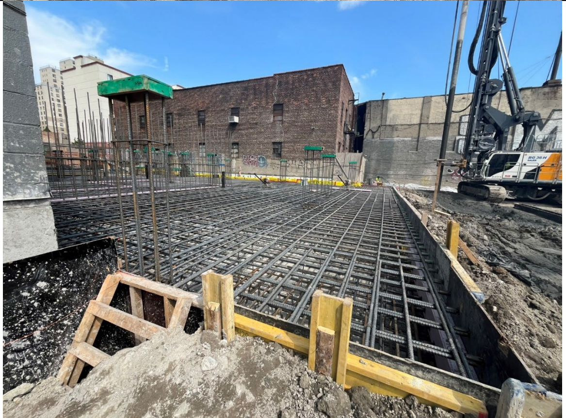
Photo 4- Representative photo of rebar work in the Butler Corridor.
