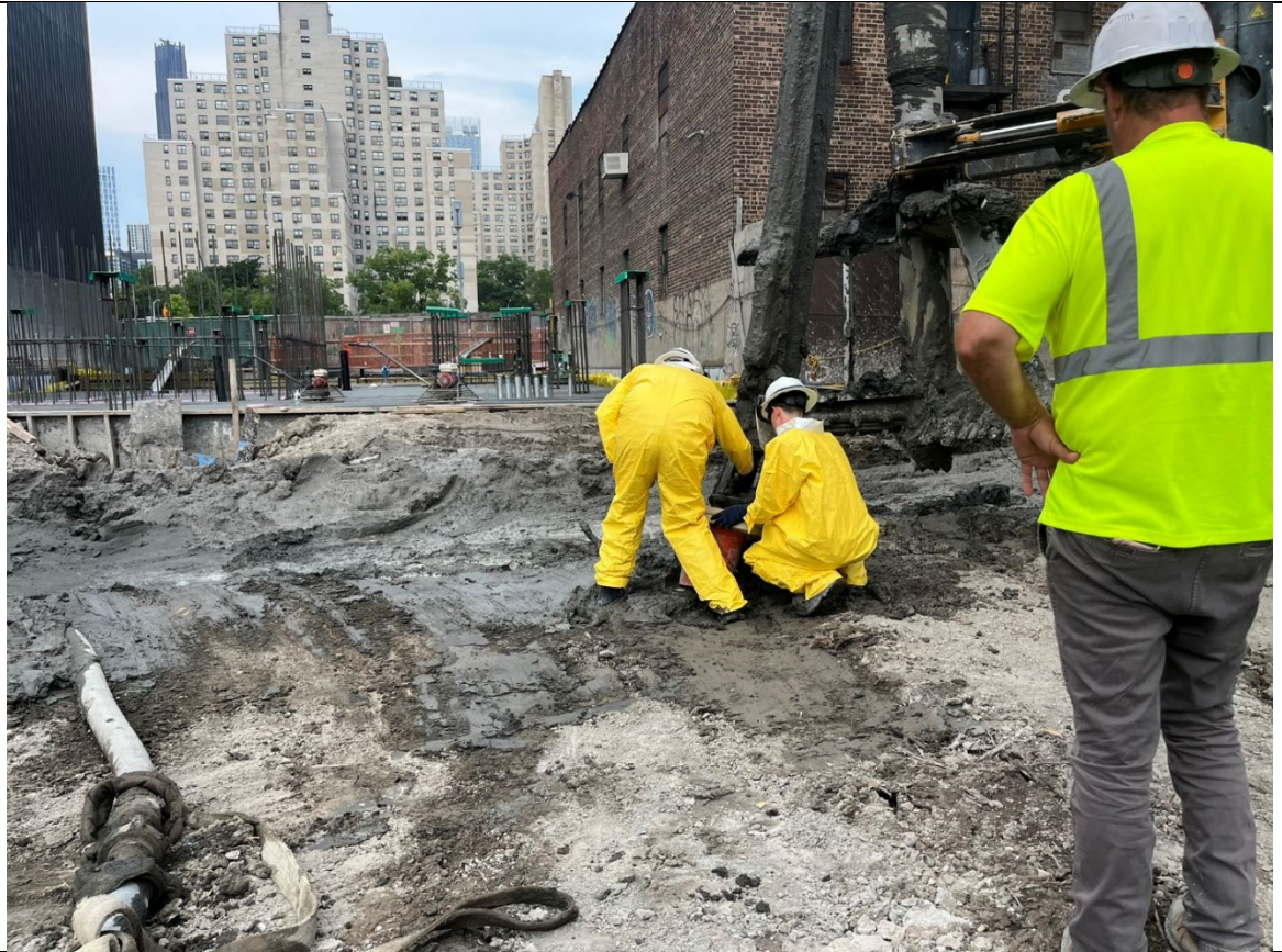
Photo 3- Representative photo of Cascade collecting a wet mix sample from Column 414 at 37.5 ft bgs.
