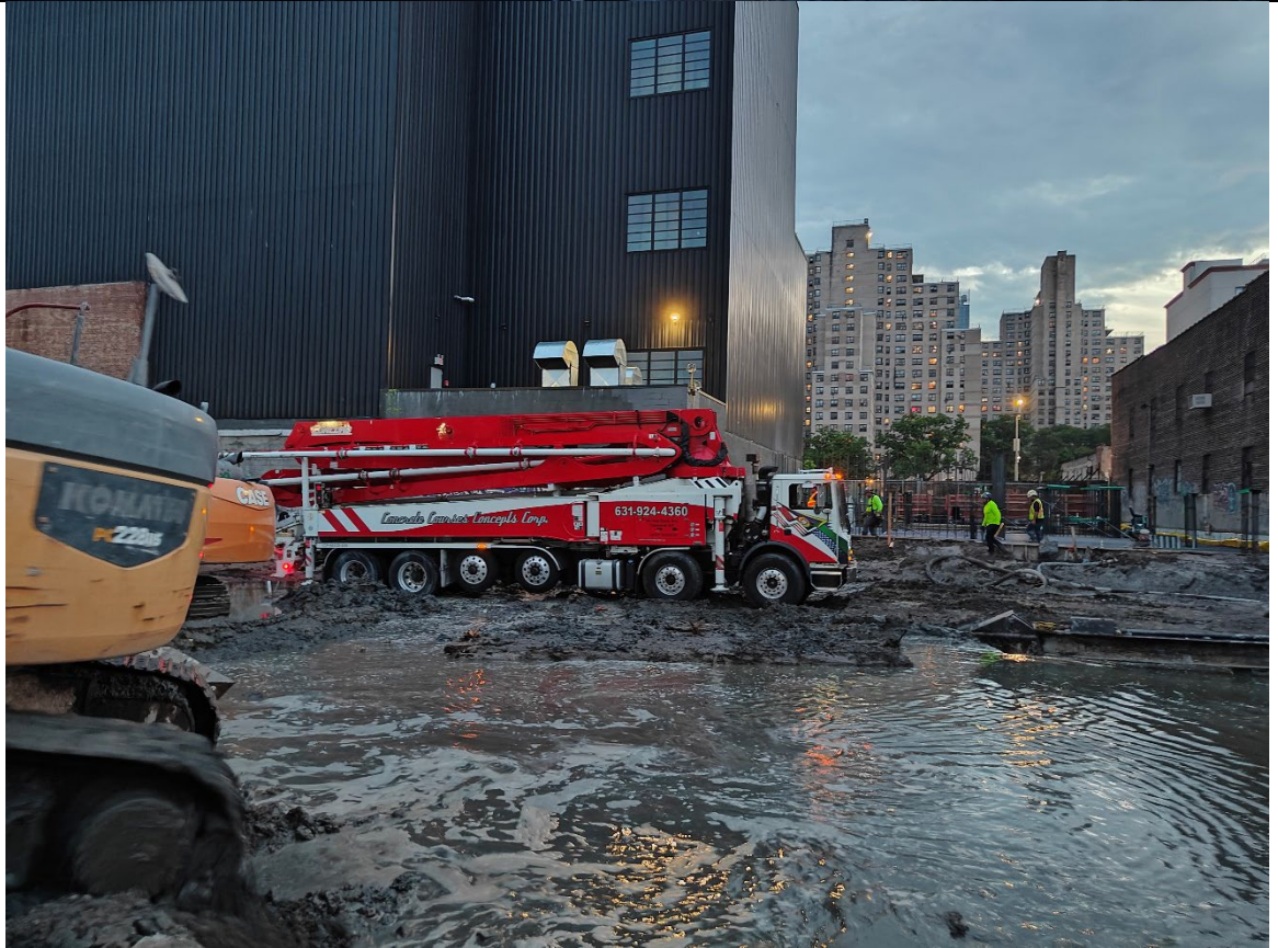
Photo 2- Representative photo of concrete pipe truck arriving on site.
