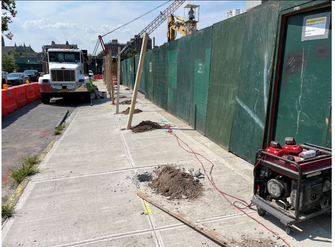
Photo 4- Representative photo of fence relocation.
