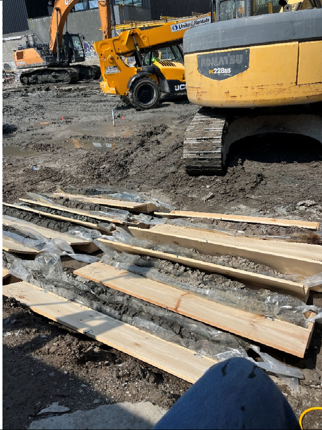
Photo 3- Representative photo of cores from core drilling.
