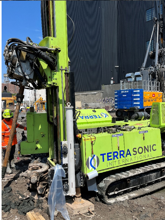
Photo 2- Representative photo of coring an ISS column.
