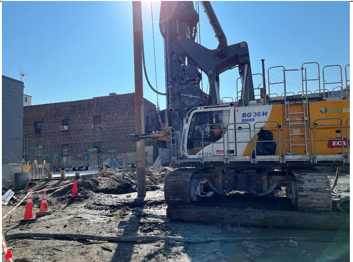
Photo 1- Representative photo of an ISS column being drilled.
