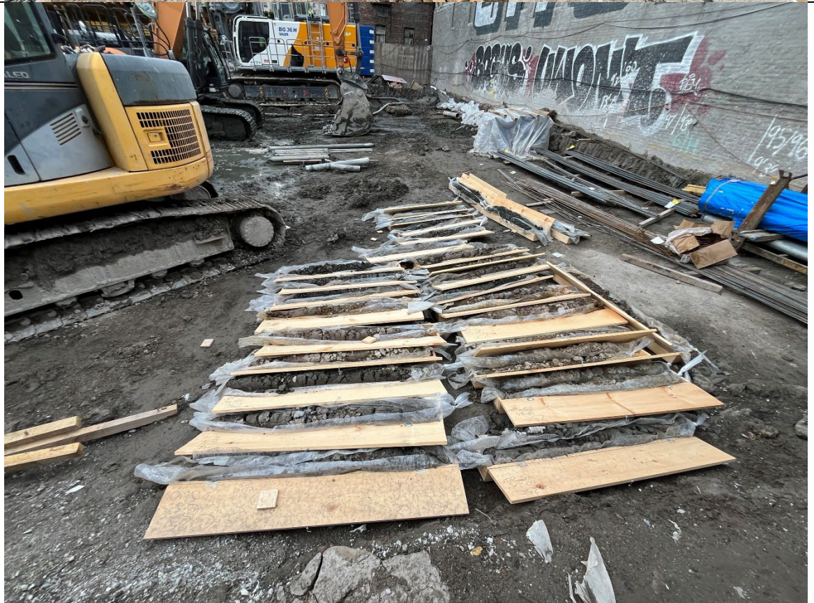
Photo 2- Representative photo of cores from core drilling.
