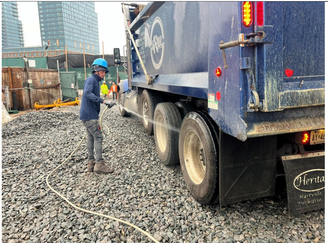
Photo 4- Representative photo of tires being washed on a truck before leaving the Site.
