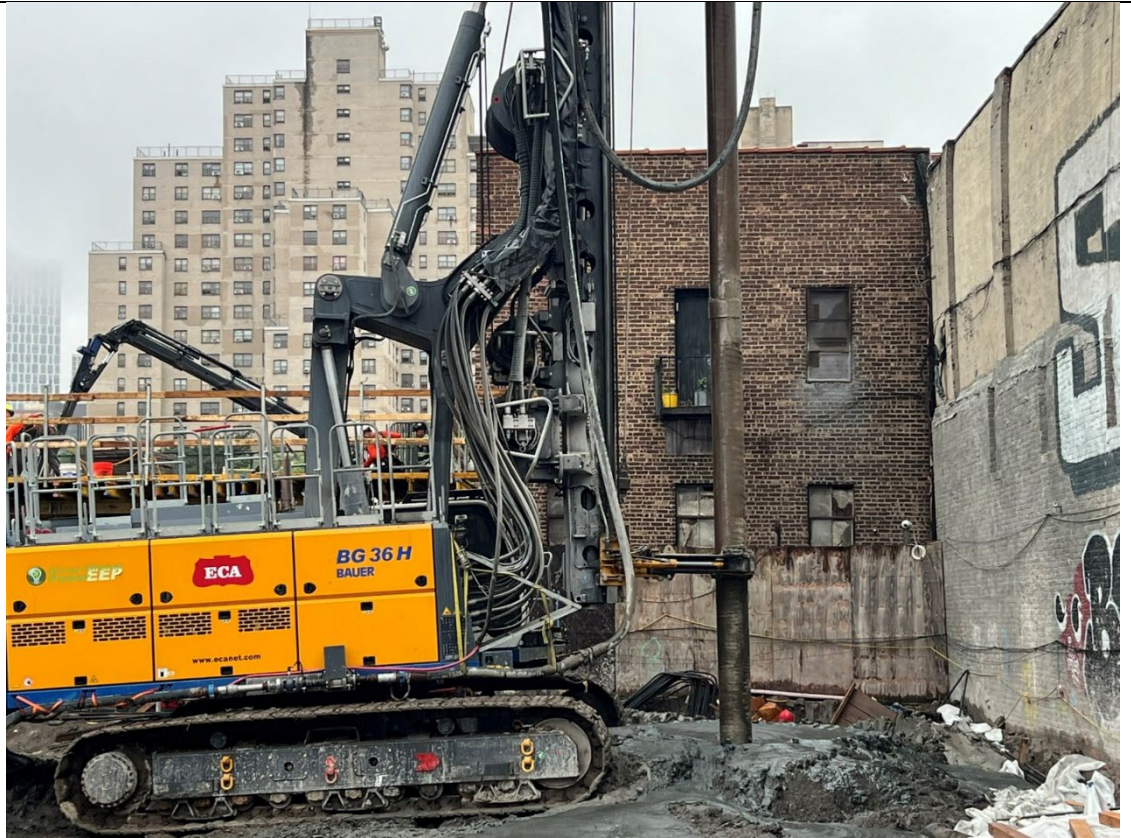
Photo 5- Representative photo of Cascade drilling an ISS column.
