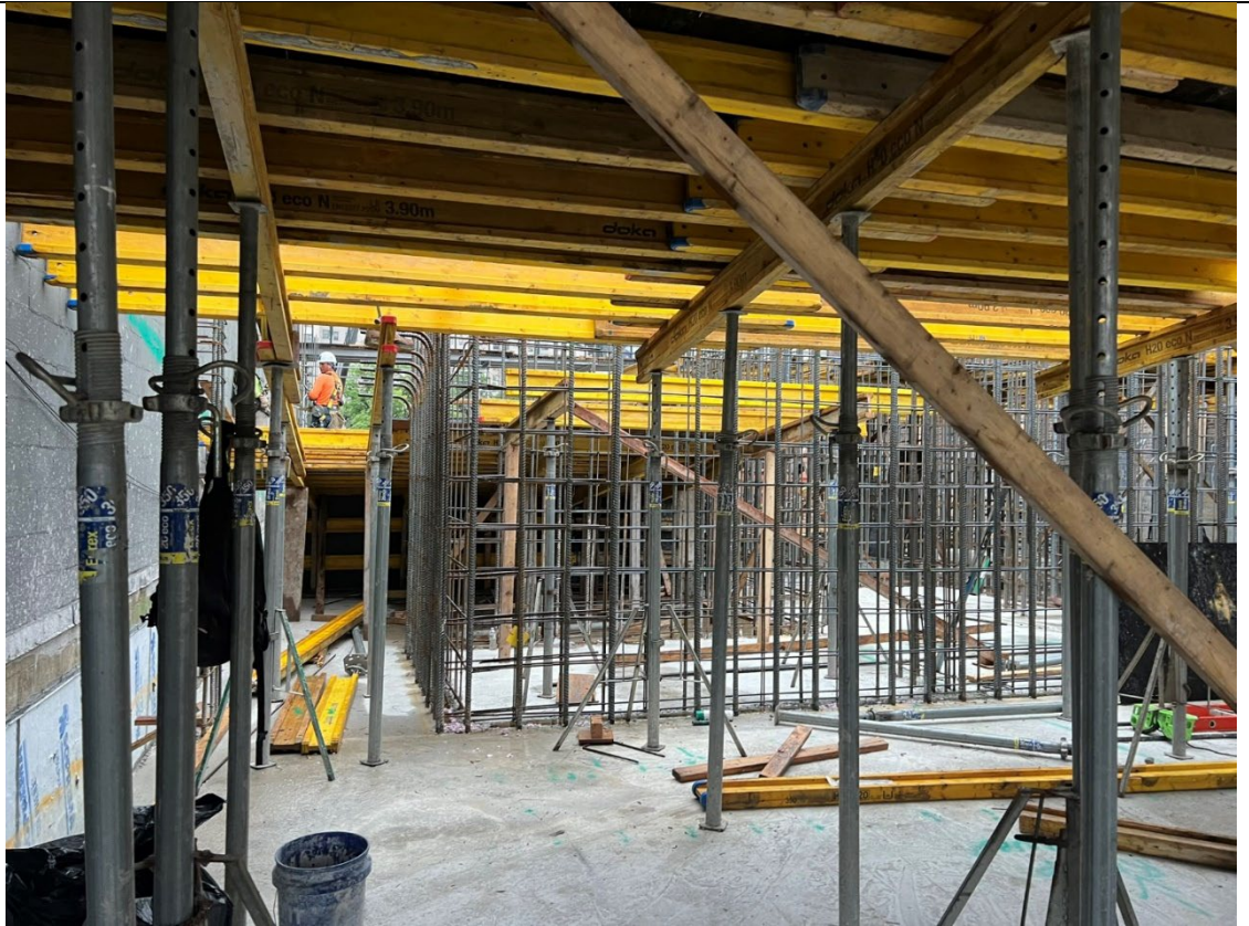
Photo 1- Representative photo of Concrete Courses continuing rebar work.
