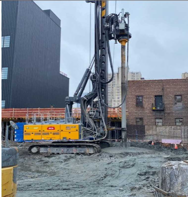
Photo 2- Representative photo of ISS column installation.
