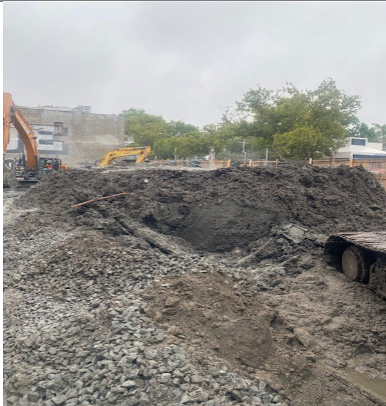
Photo 3- Representative photo of swell material consolidated into a stockpile.
