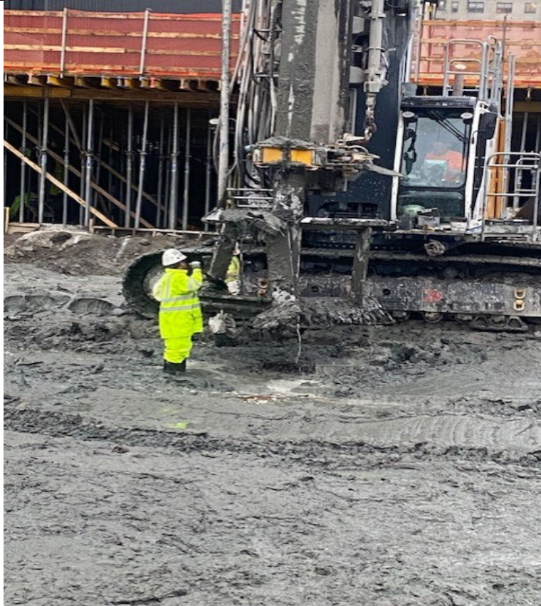
Photo 5- Representative photo of crew cleaning debris from auger at end of shift.
