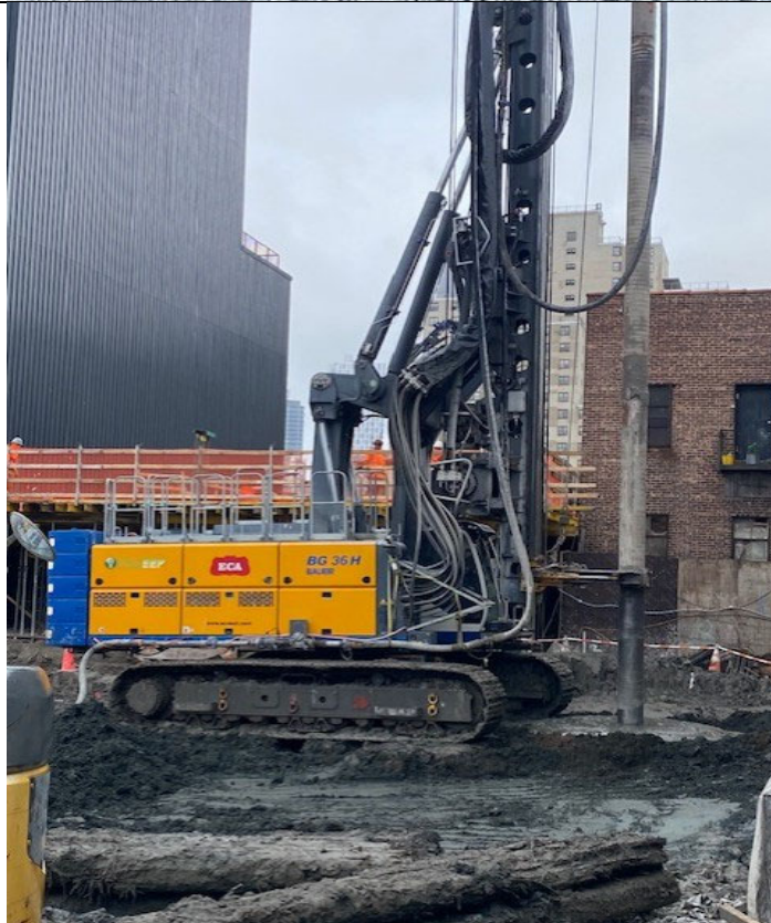
Photo 2- Representative photo of ISS column installation.
