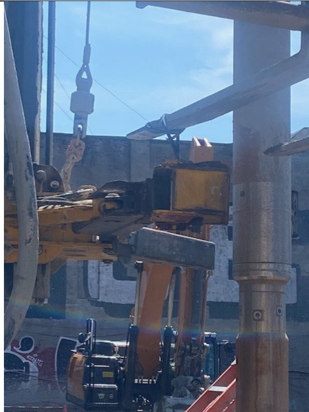
Photo 5- Representative photo of Cascade re-installing repaired centralizer to ISS drill-rig.
