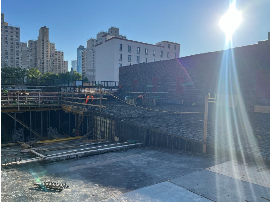
Photo 4- Representative photo of rebar in northern corridor.
