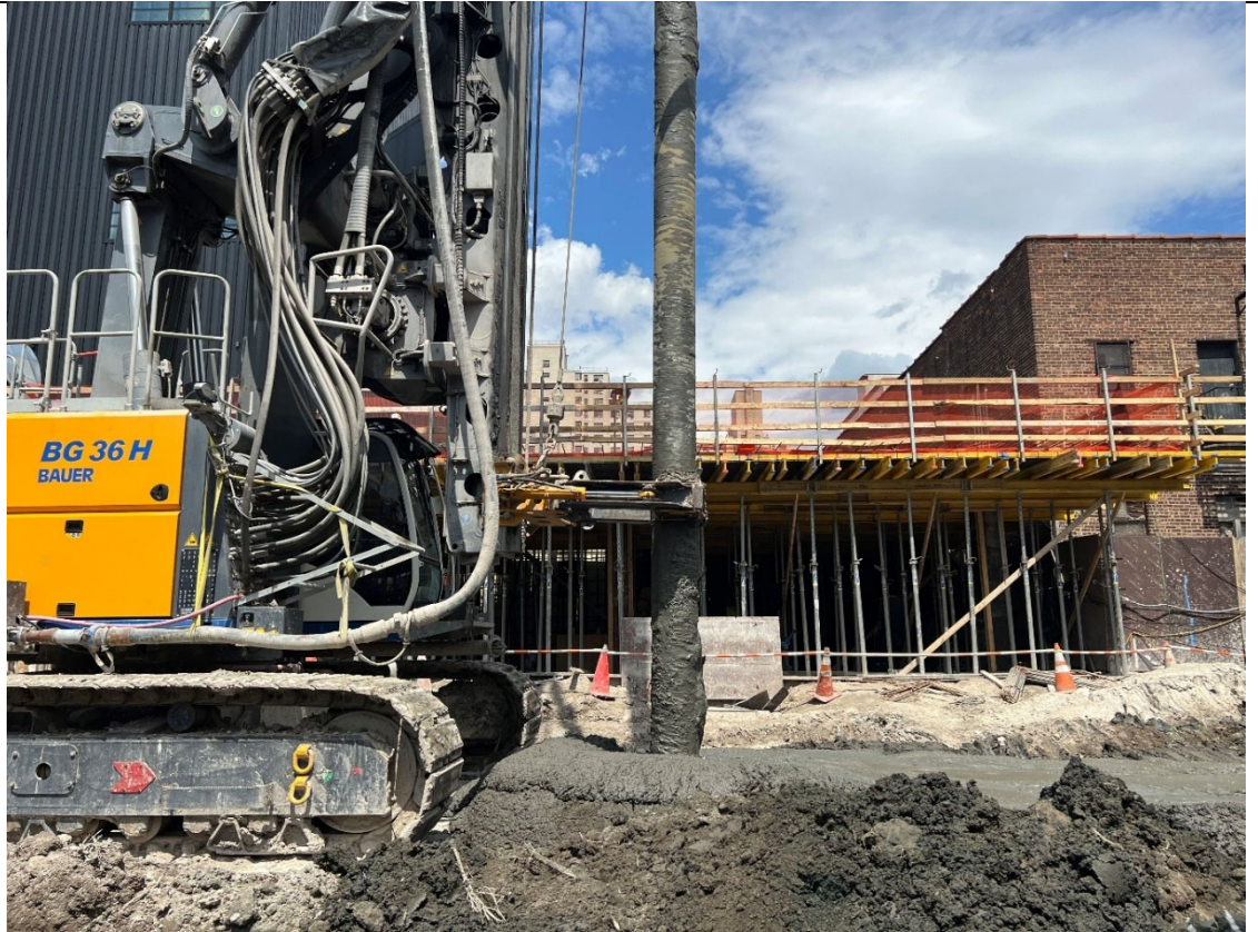
Photo 1- Representative photo of ISS column installation.
