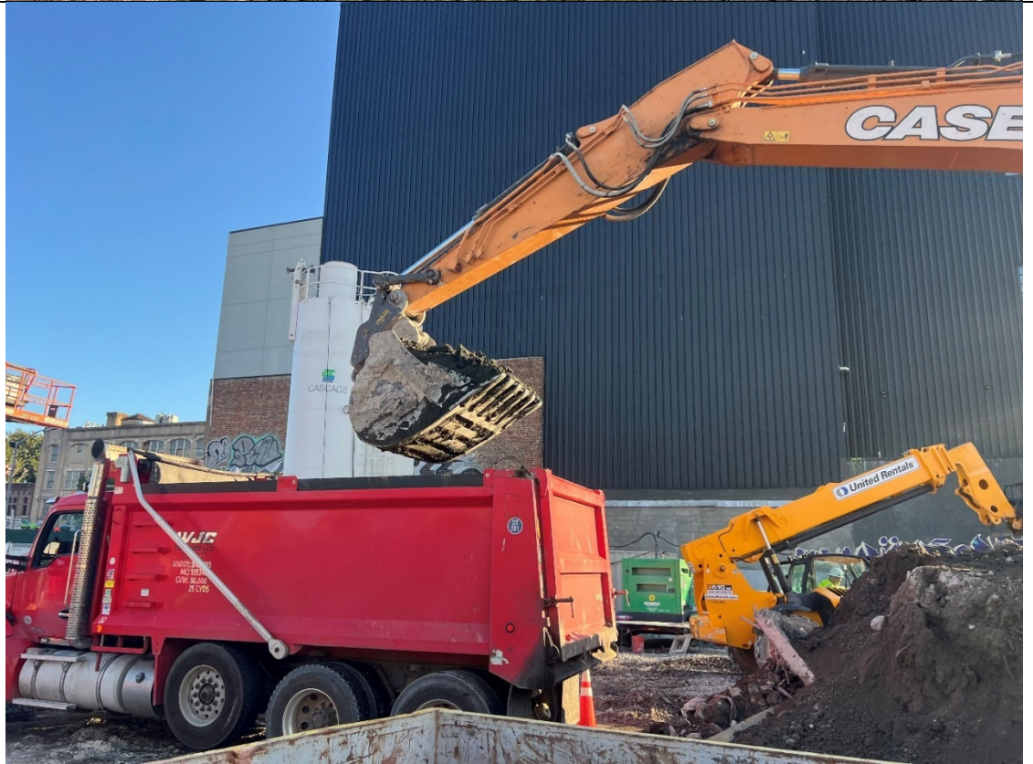
Photo 2- Representative photo of swell material trucking.
