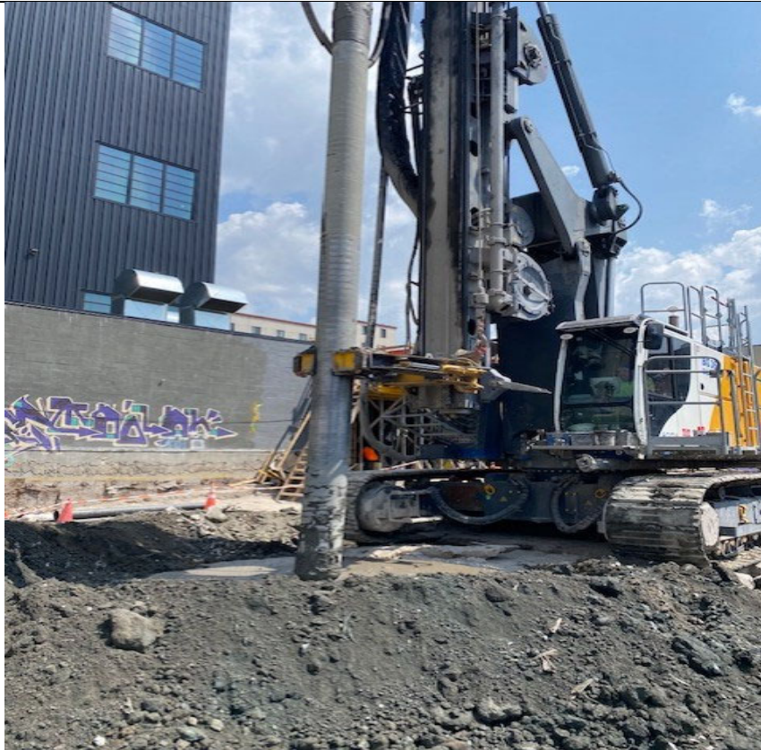
Photo 1- Representative photo of ISS column installation.
