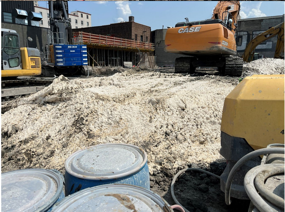
Photo 2- Representative photo of ATMOS foam applied to swell material.
