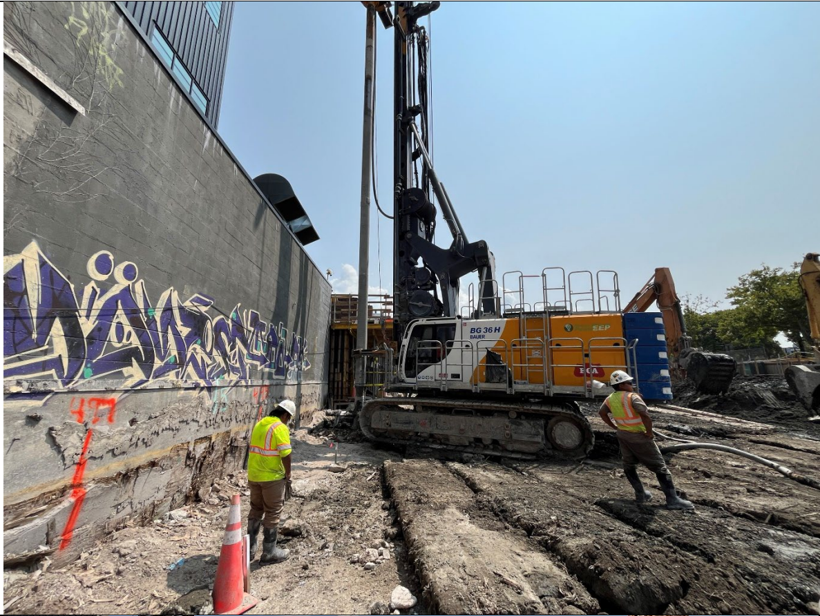
Photo 1- Representative photo of ISS column installation.
