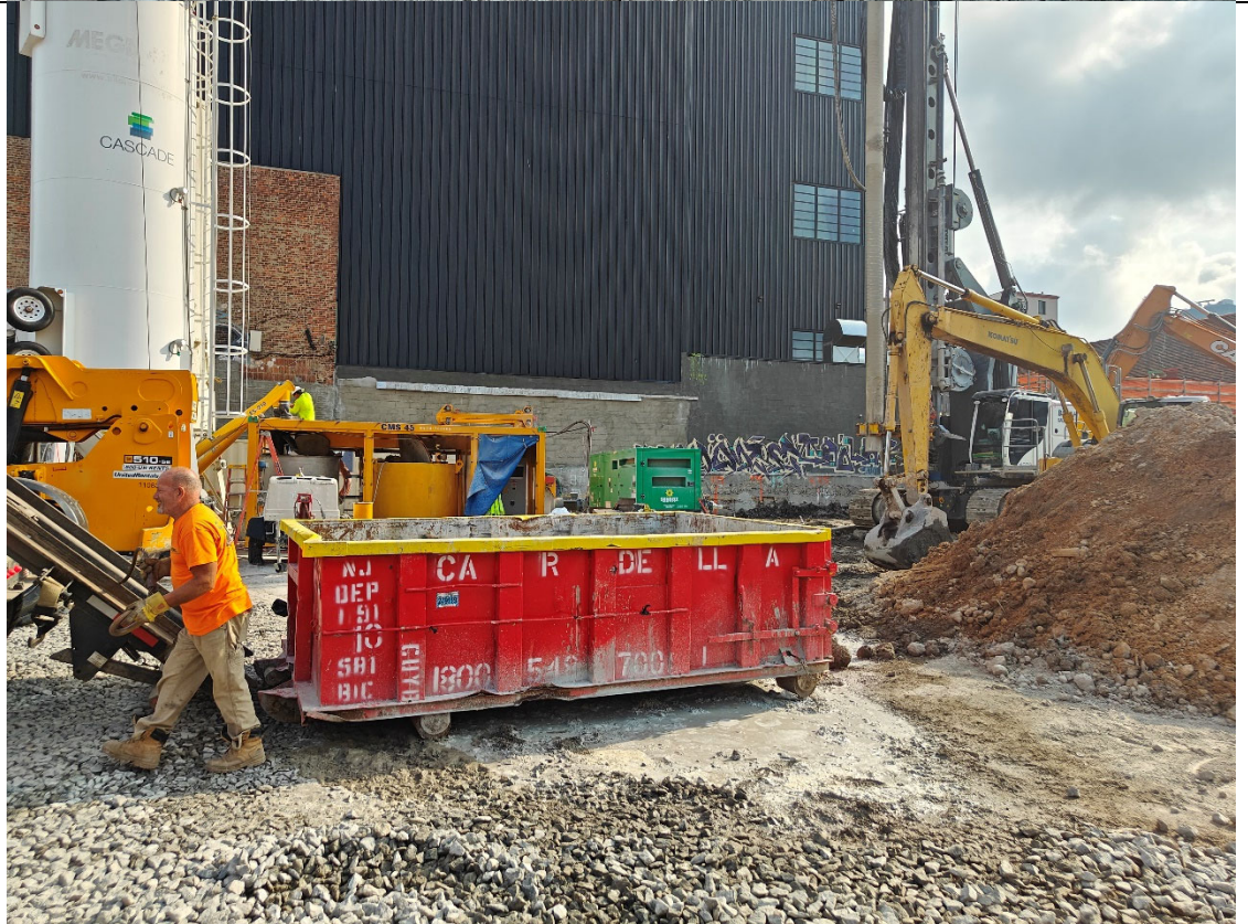
Photo 2- Cardella replaces rolloff container.
