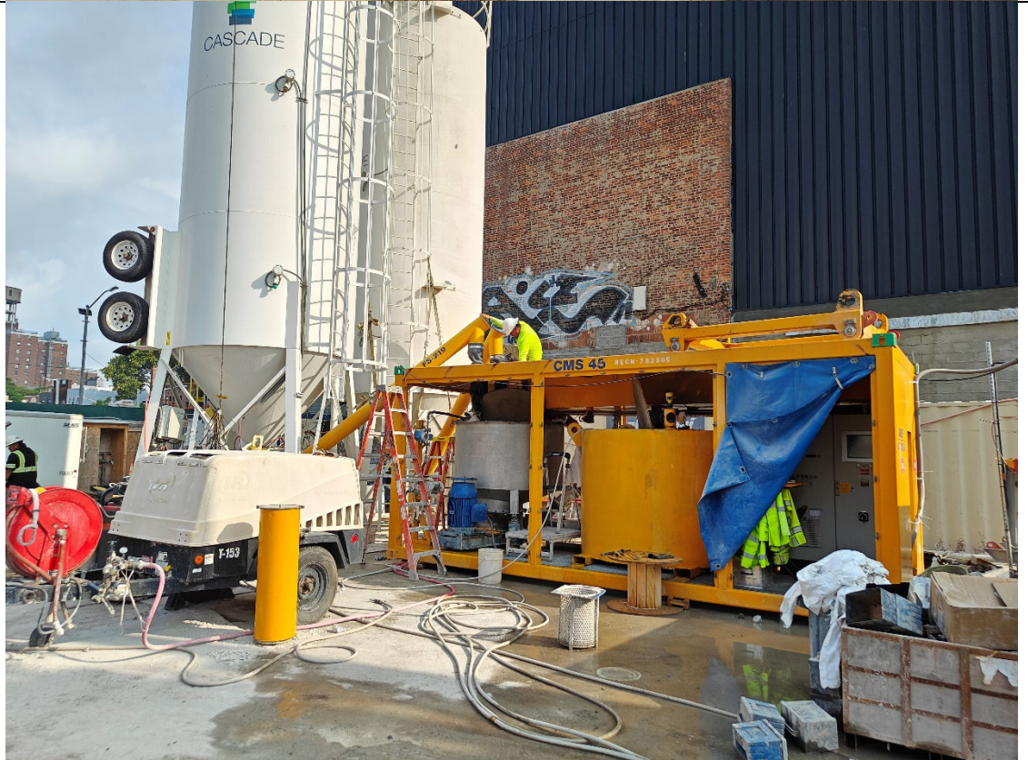
Photo 4- Representative photo of batch plant maintenance.
