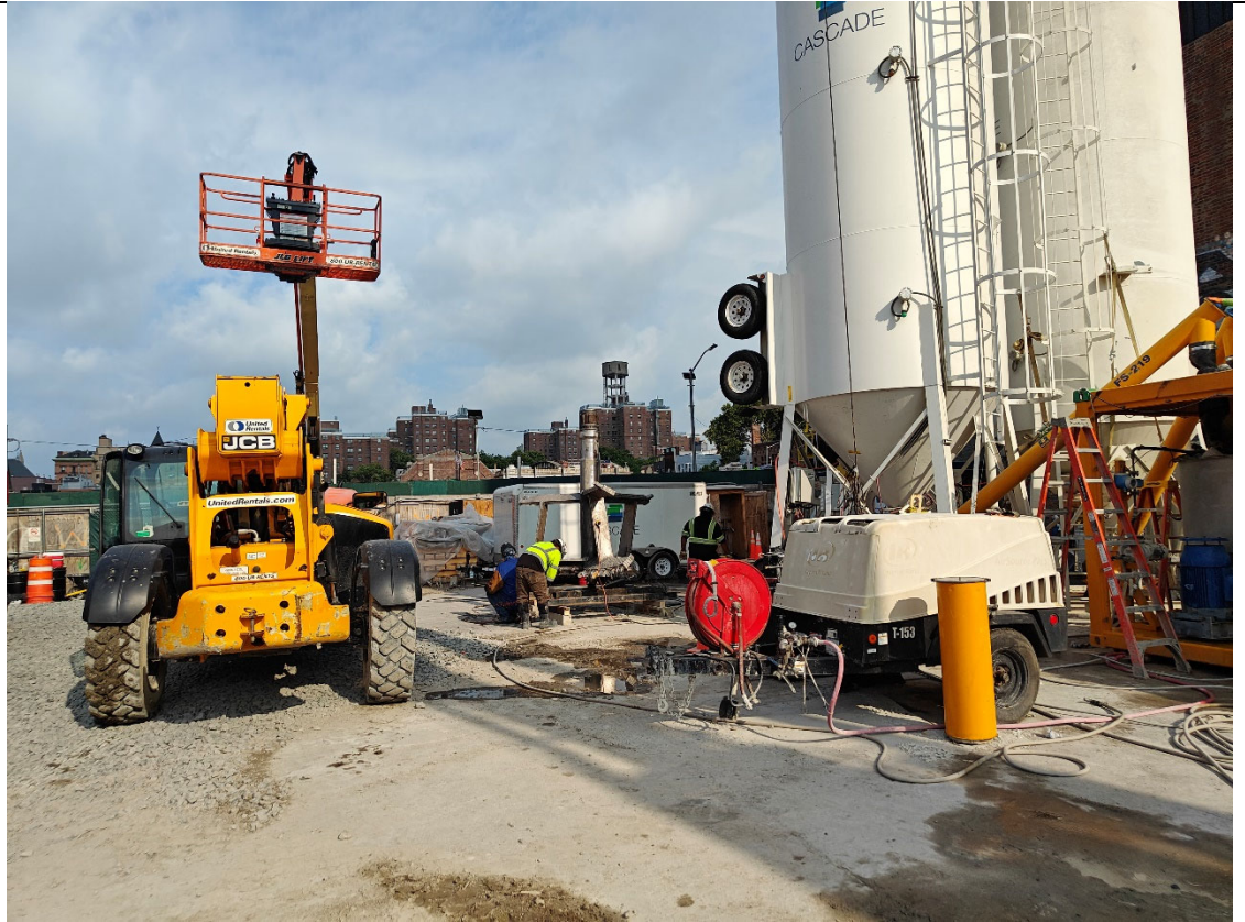
Photo 3- Representative photo of augur maintenance.
