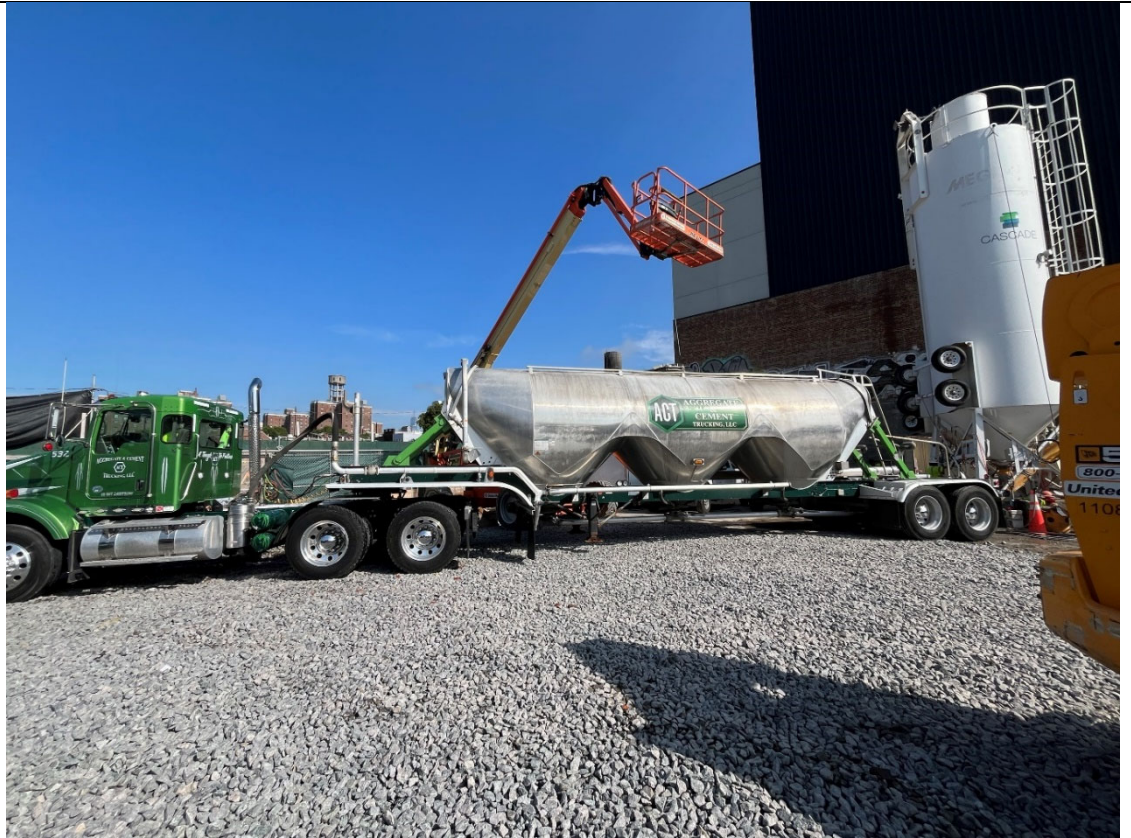
Photo 3- Representative photo of slag delivery.
