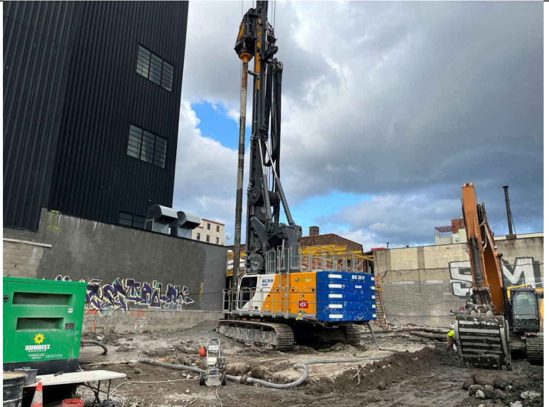
Photo 1- Representative photo of ISS column installation.
