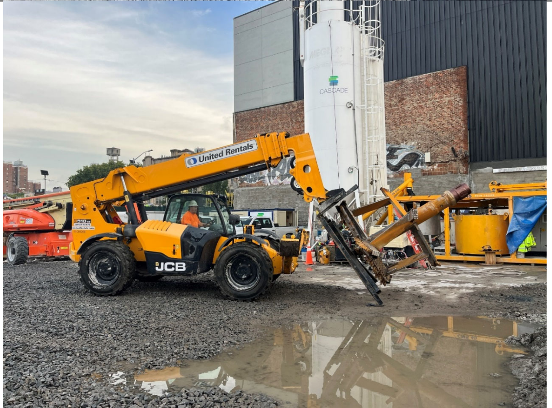
Photo 4- Representative photo of auger being reattached to the Kelly Bar.
