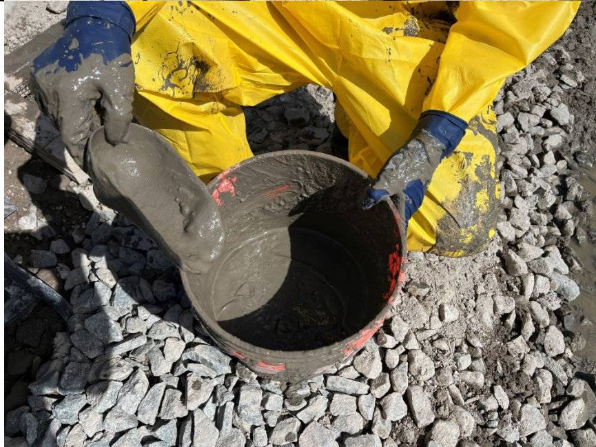
Photo 2- Representative photo of wet mix sample collected from column 399.
