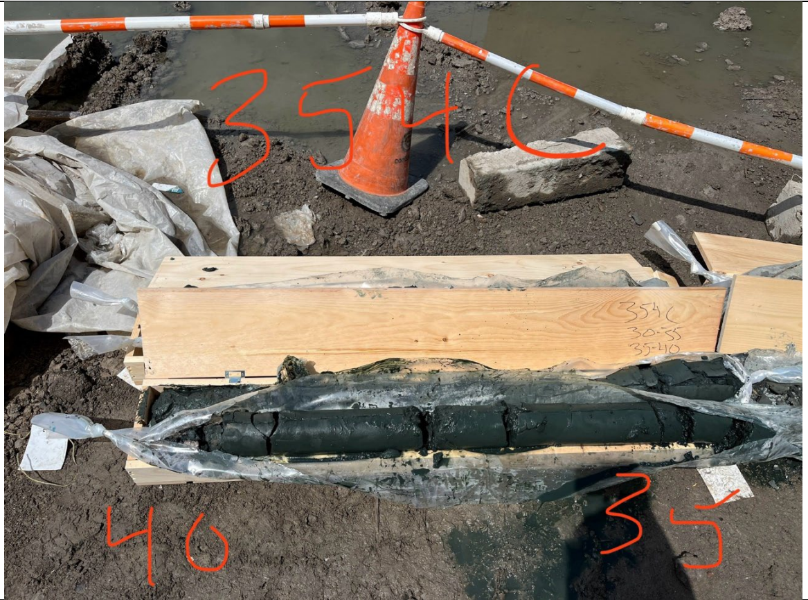
Photo 3- Representative photo of QA/QC cores.
