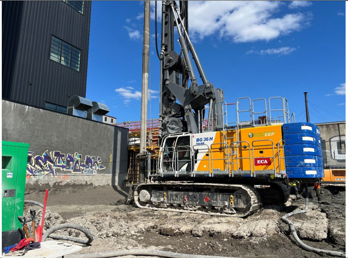
Photo 1- Representative photo of ISS column installation.
