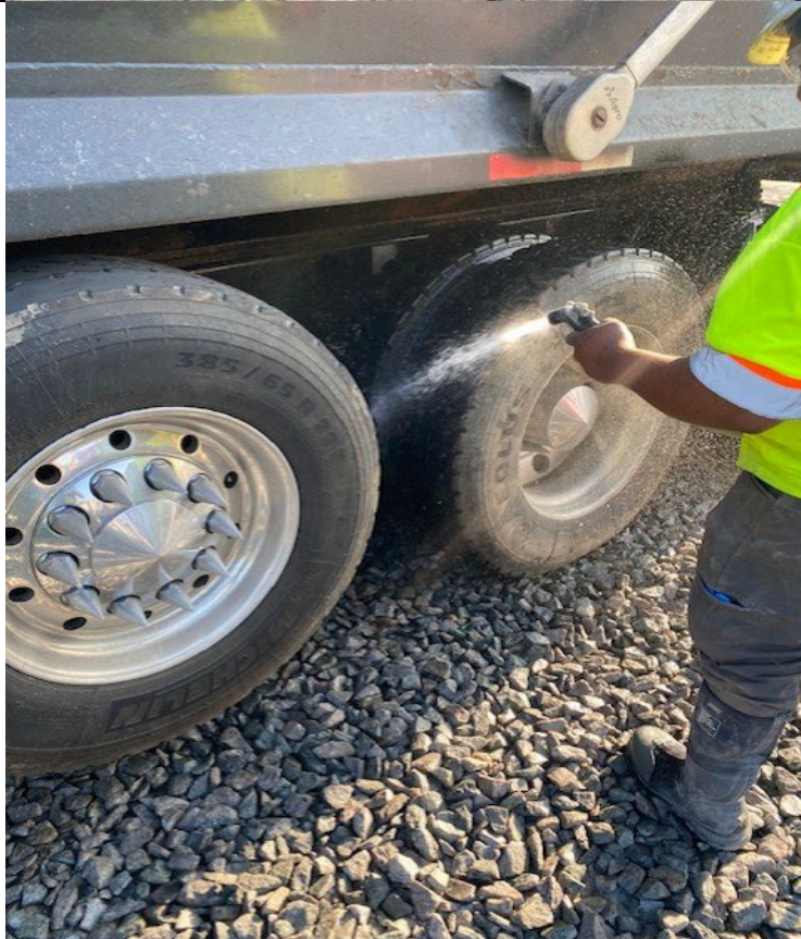
Photo 2- Representative photo of Cascade crew washing wheels of each truck departing Site over track pad.
