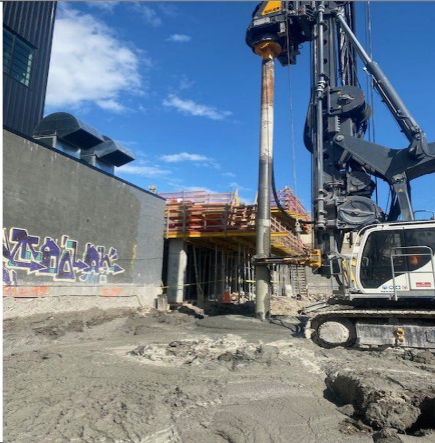
Photo 1- Representative photo of ISS column installation.
