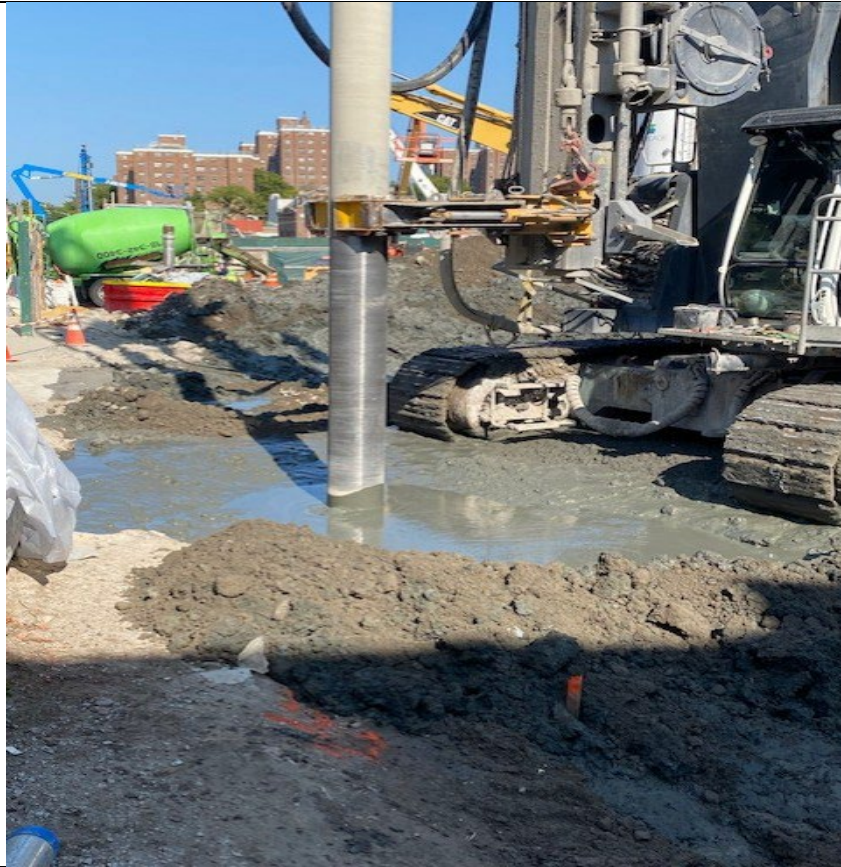
Photo 1- Representative photo of ISS pilot column over-drill with 6' auger.
