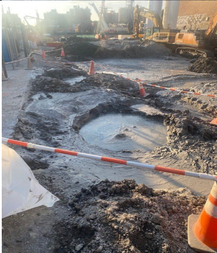
Photo 2- Representative photo of completed over- drilled columns 23 and 25.
