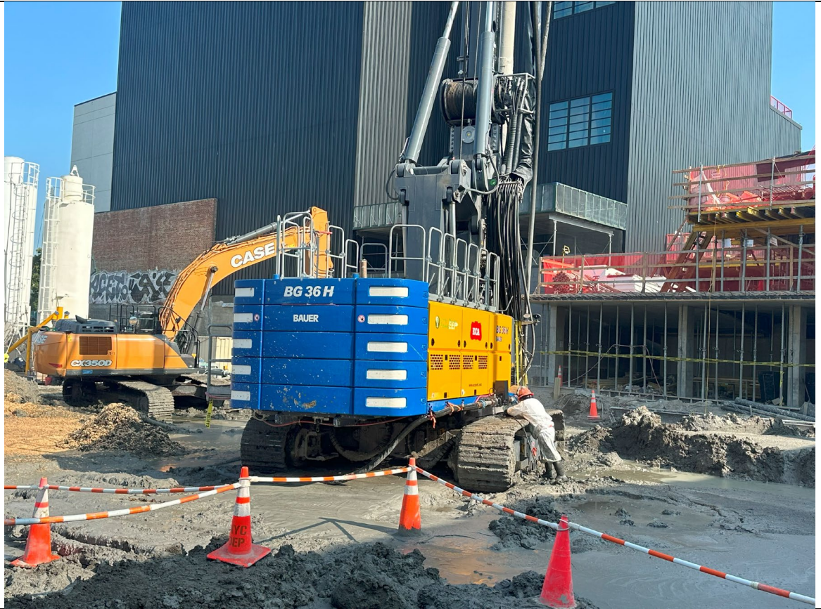
Photo 3- Representative photo of rig maintenance.
