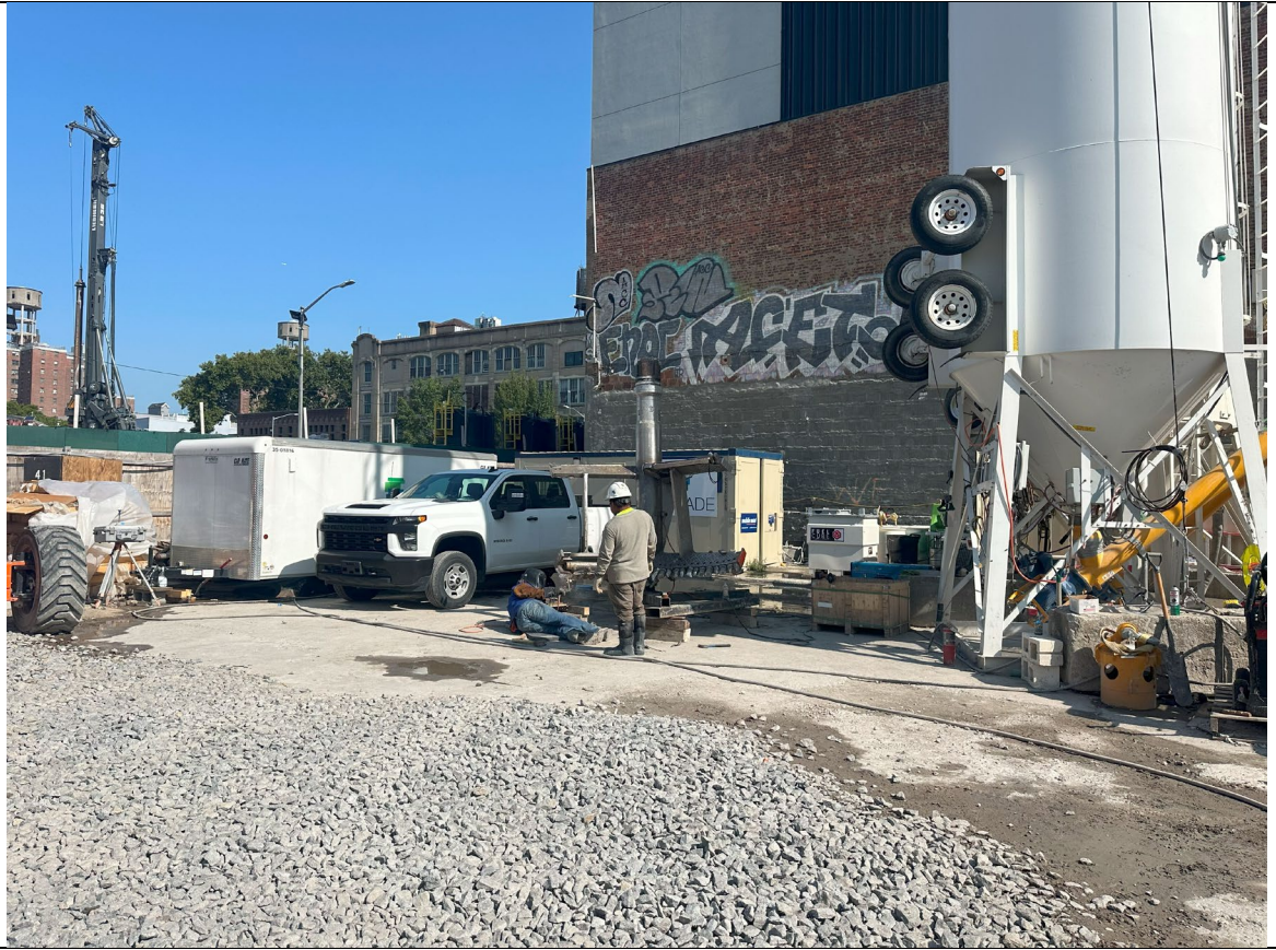
Photo 5- Representative photo of rig auger being welded.
