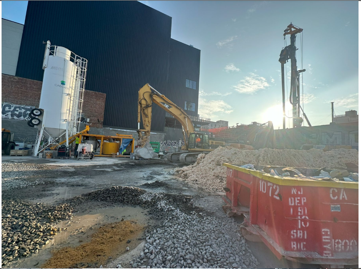
Photo 1- Representative photo of batch plant maintenance.
