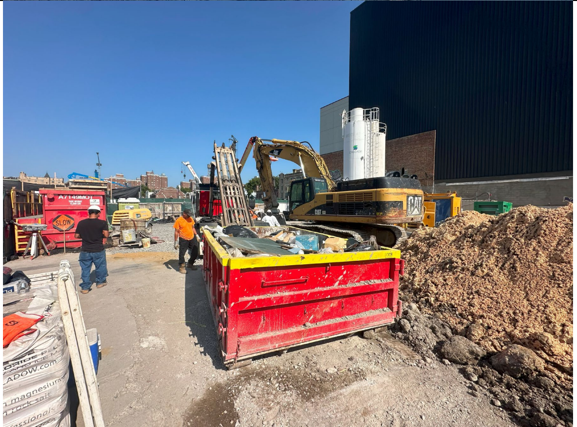
Photo 4- Representative photo of Cardella replacing Rolloff container.
